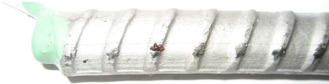
Figure 14: Coiled XM-28 stainless steel from producer A after testing; specimen XM28c-1. Anode bar with limited corrosion products at a damage site.
