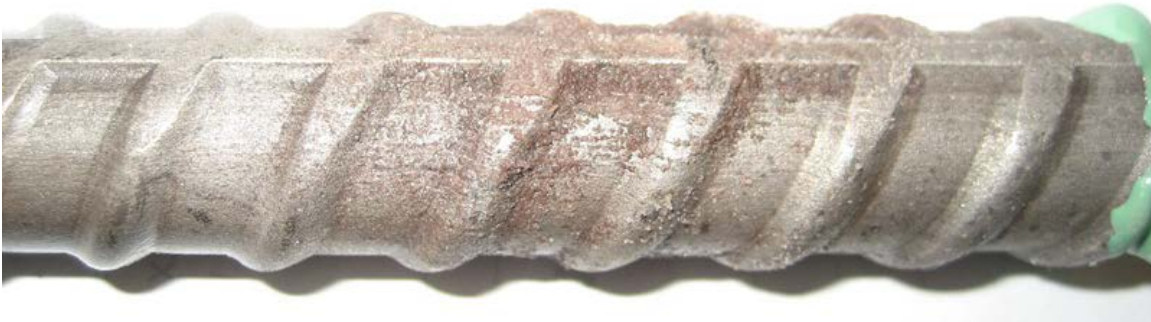
Figure 20b: 2205 stainless steel from producer B showing closeup of corrosion products after testing; specimen 2205-3.
