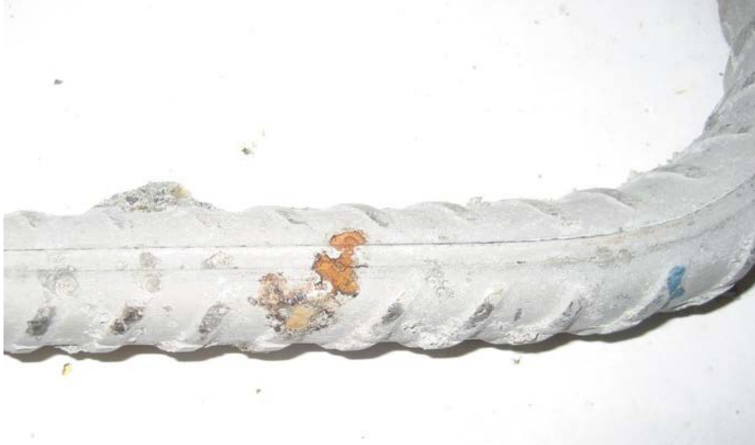
Figure 80a: Corrosion staining on SSClad-b-2 upon autopsy, bent NX-SCR™ stainless steel clad bar (close-up)
