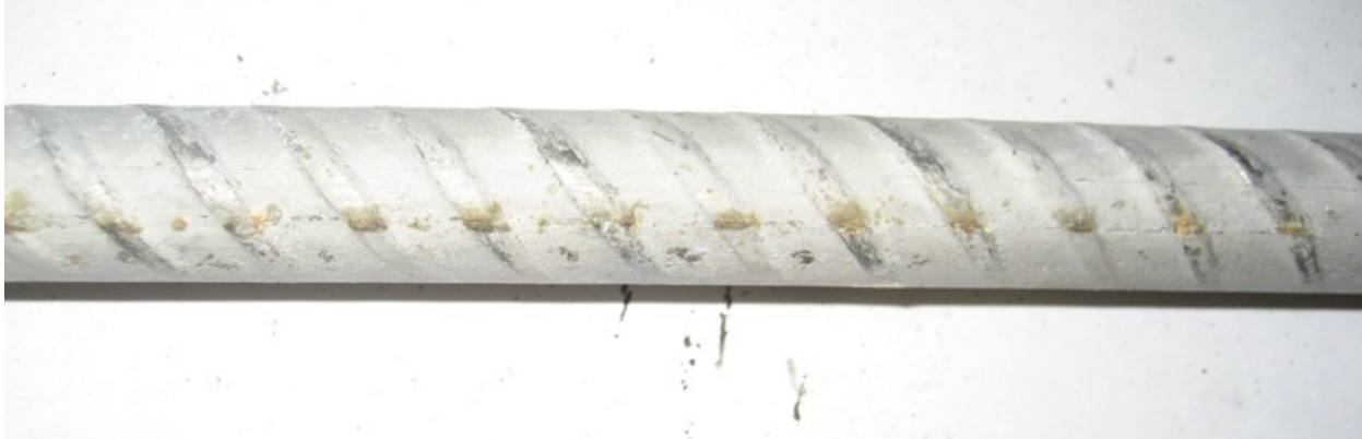
Figure 77a: CB-SSClad-1 top bar upon completion of test showing corrosion on deformations
