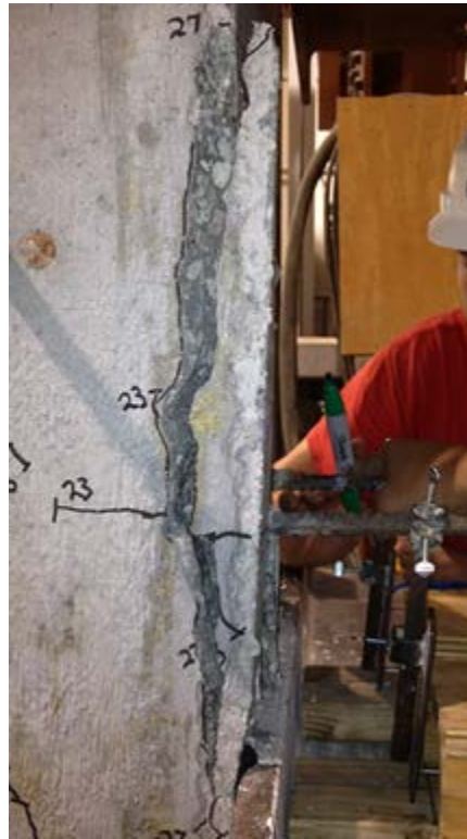
Figure 8 Front pullout failure
