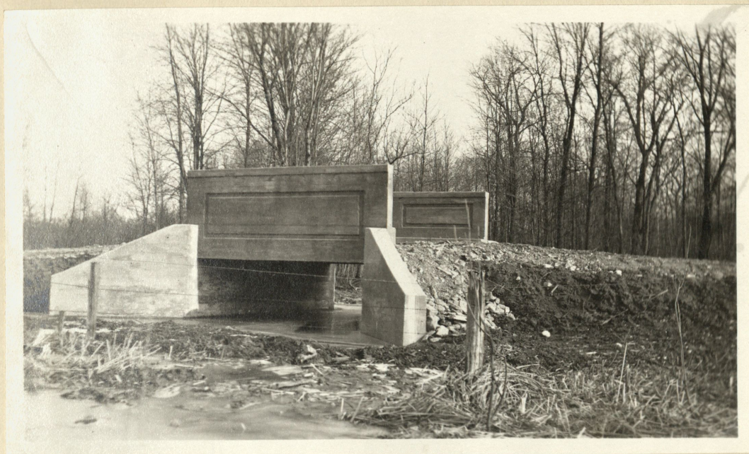
Reinforced concrete Bridge of Flat Slab type. Town of Hortonia, Outagamie County. Span 12 feet, Roadway 20 feet, Cost $600.
