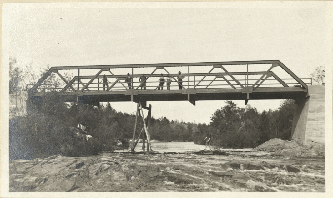
Morrison Creek Bridge, Town of Brockway, Jackson County. A typical pony truss, span 80 feet, Roadway 16 feet. Cost $3323.
