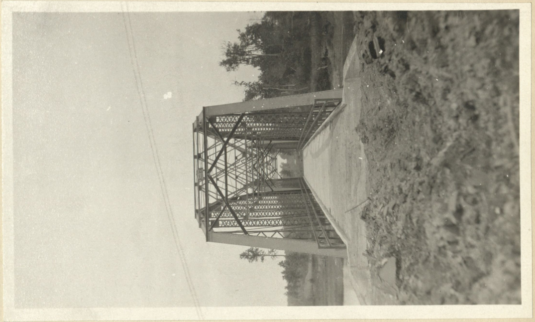
Fisk Bridge, Town of Holcombe, Chippewa County. Two curved chord Pratt trusses; Span 140 feet; Roadway 16 feet; Cost $10274.
