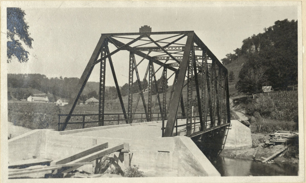
Simmons Bridge, Town of Forest, Richland County. A typical High Truss: Span 90 feet, Roadway 16 feet. Cost $3950.
