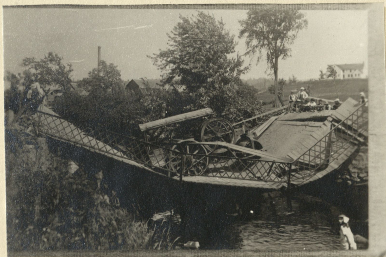
A typical failure under a traction engine. Nobody was hurt.
