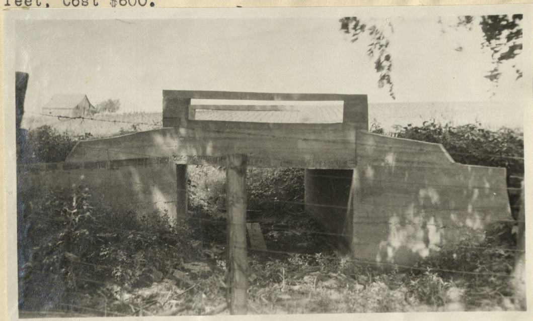
The result of an incompetent builder. Gates Bridge, Town of Beetown, Grant county, built by local authorities without supervision. Span 10 feet, Roadway 20 feet; Cost $330.
