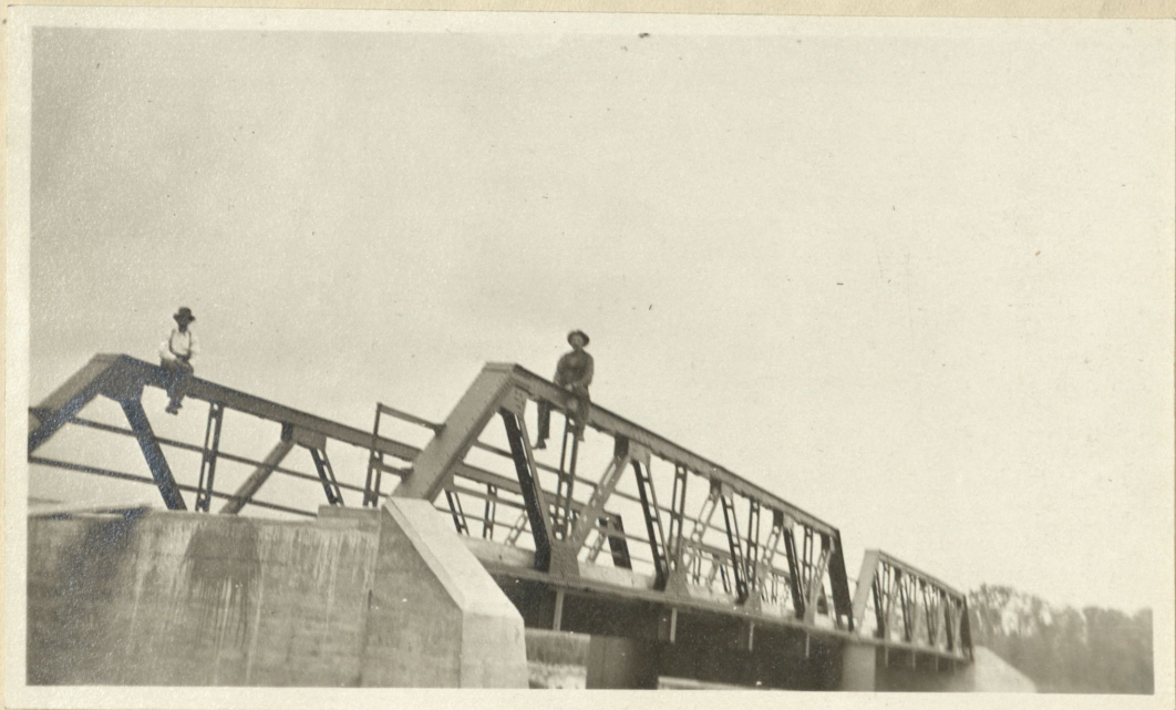
Tichigan Bridge, Town of Waterford, Racine County. Two 70 feet spans, 16 feet roadway, Pony trusses. Mass con- crete abutments and Tubular pier. Cost $4104.
