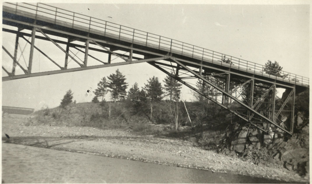
Hatfield Bridge, Town of Brockway, Jackson County. A three hinged Arch. Span 180 feet; Roadway 16 feet. Two approach spans of 20 feet. Fifty feet above streambed at center of span. Cost $4950. Built under Commission's supervision in 1912.
