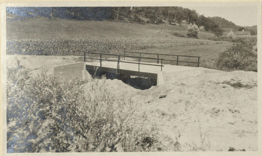
Dalberg Bridge, Town of Akan, Richland County. A typical I-Beam bridge; span 28 feet; Roadway 16 feet. Cost $1200.
