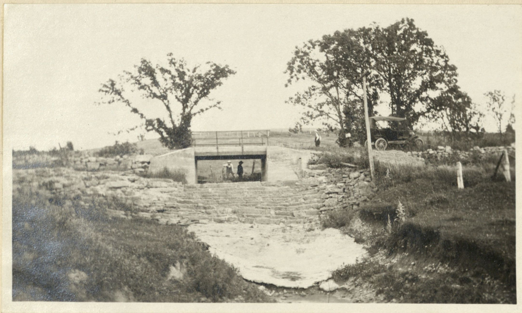
Sutters Bridge, Town of Paris, Grant County. An I-beam bridge with well réprapped streambed. Span 16 feet; Roadway 16 feet. Cost $571.
