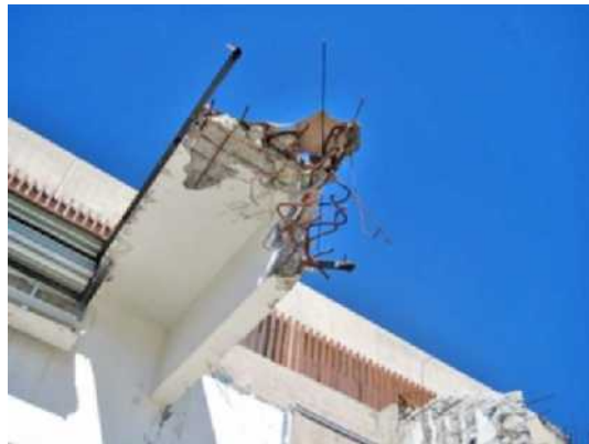
Figure 12. Pilaster at axes A and 11 (top of the first story), 29 November 2010.
