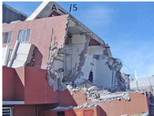
Figure 8. Wall along axis 5, 29 March 2010. Photo credit: G. Alarcón.
