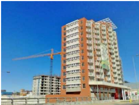
Figure 1. The Alto Río Building before collapse (view from northwest). Taken from http://www.chw.net/foro/off-topic-fl6/309633-edificio-alto-rio-Concepcion-antes-despues.html .
