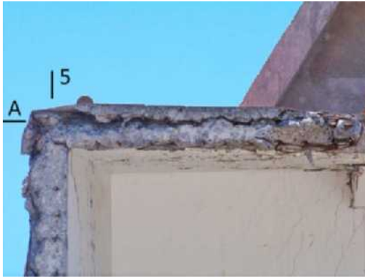
Figure 9. Splitting cracks in wall segments.
