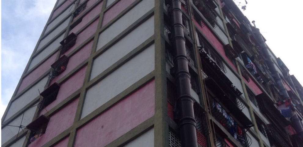
Figure V-1 Trash chutes were recently replaced in 23 de Enero
