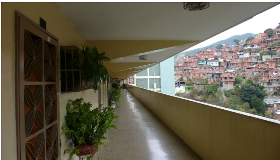
Figure IV-14 Open corridor in the twelfth level of Cerro Grande. The picture is taken close to the north circulation tower looking toward the south one. The door in the foreground is that of a 3-Bedroom apartment. 4-bedroom apartments in the upper level are accessible from this corridor using staircases.
