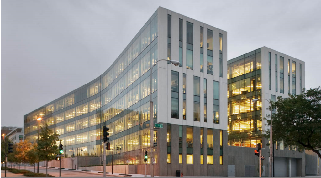
Figure 7.1: JE Dunn Headquarters Building
