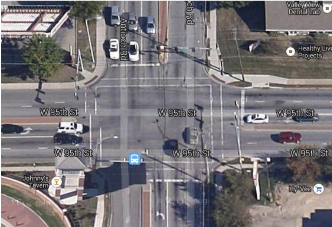
Figure 53. 95th Street and Antioch Road (aerial image, Google Earth, 2013)
