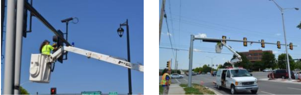
Figure 69. Field installation of the confirmation light
