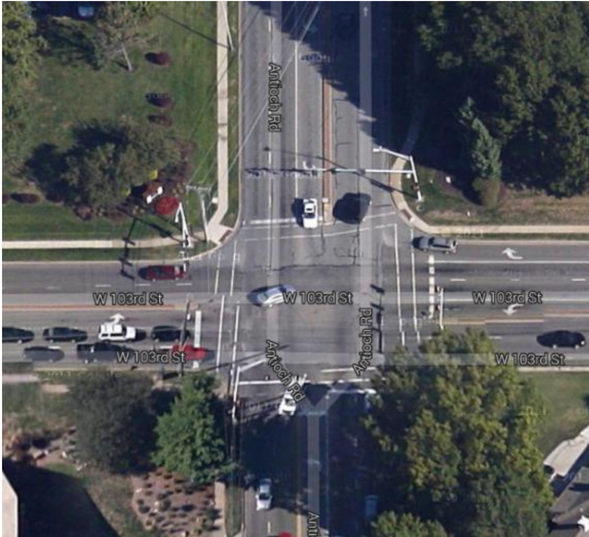
Figure 56. 103 rd Street and Antioch Road (aerial image, Google Earth, 2013)
