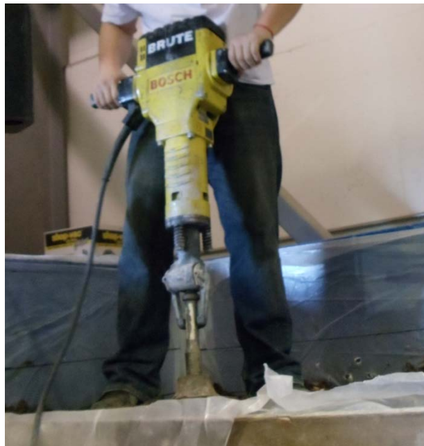
FIGURE 4.14 Compaction of surrounding soil using the jackhammer
