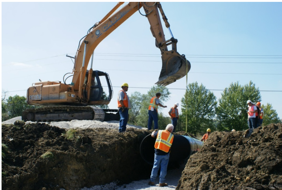
FIGURE 5.16 Placing a pipe in the trench
