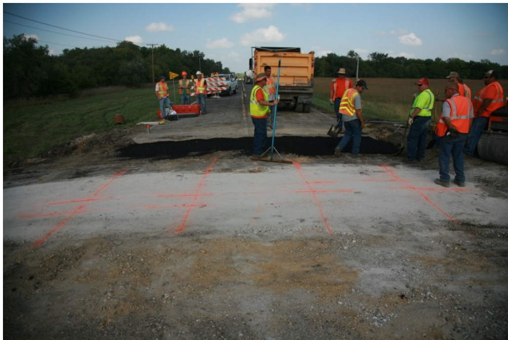
FIGURE 5.21 The compacted AB-3-II surface before placing the HMA base
