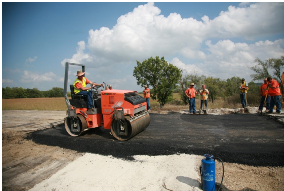
FIGURE 5.28 Vibratory roller compacting the HMA base
