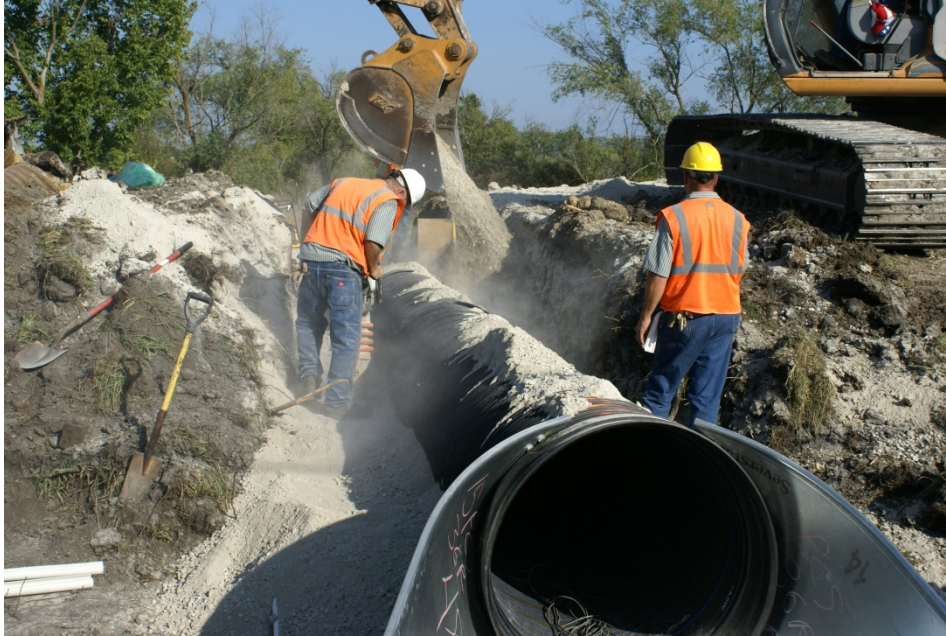
(b) Western test section (Section A)
