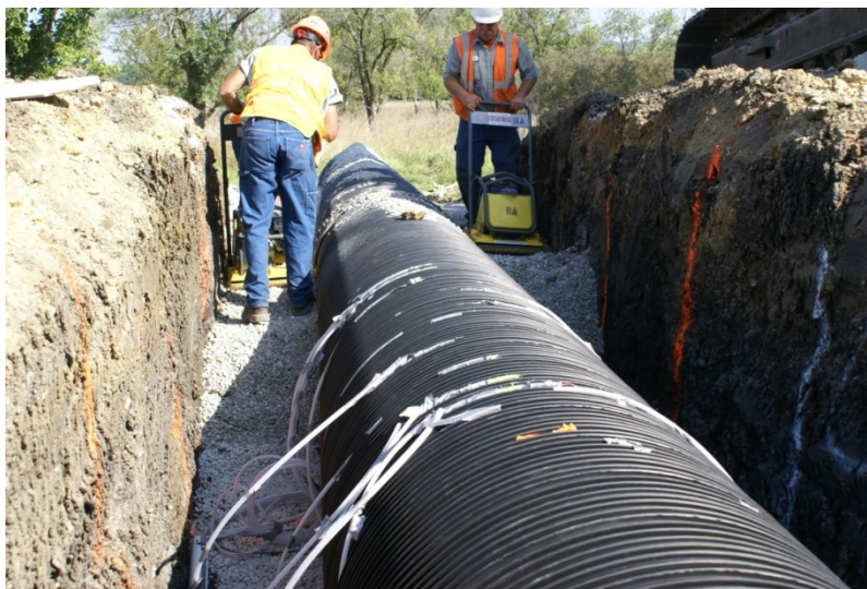
(a) Eastern test section (Section B)
