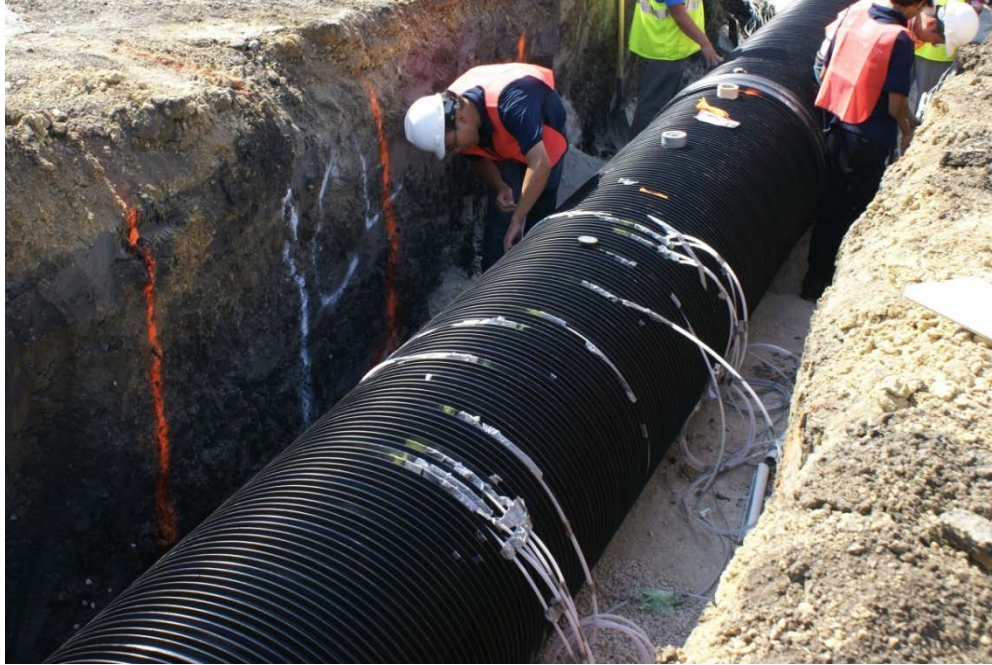
FIGURE 5.6 Strain gages fixed outside of the pipe in the field
