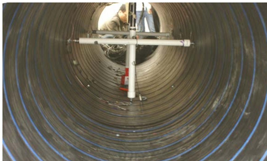
FIGURE 5.5 Displacement transducers inside the pipe section in the field
