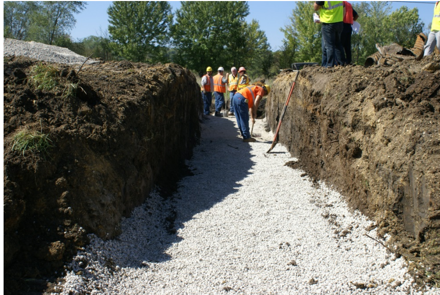
FIGURE 5.12 Construction of the beddings
