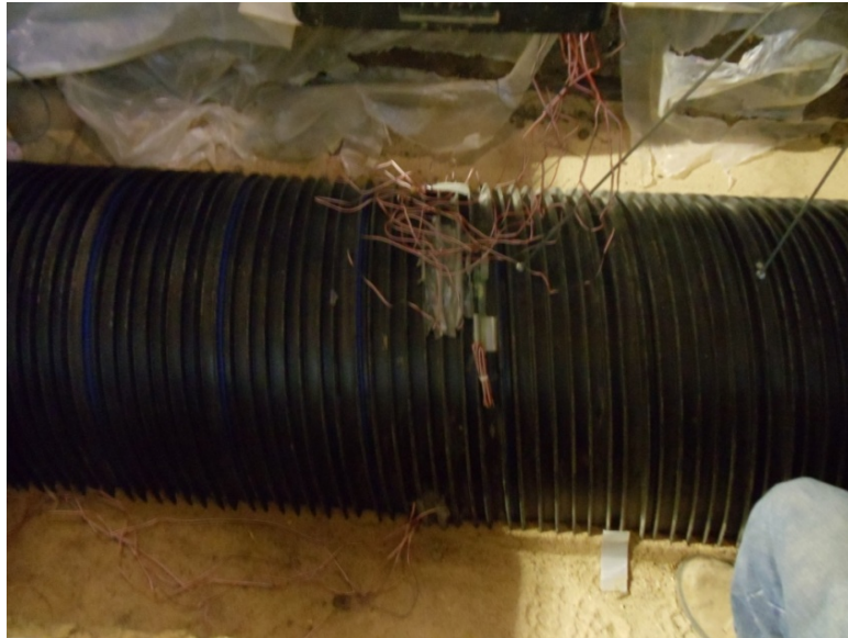
FIGURE 4.18 Backfill up to the springline in Test Section 1
