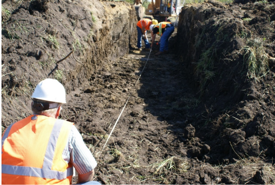
FIGURE 5.11 Marking centerline before dumping bedding materials.
