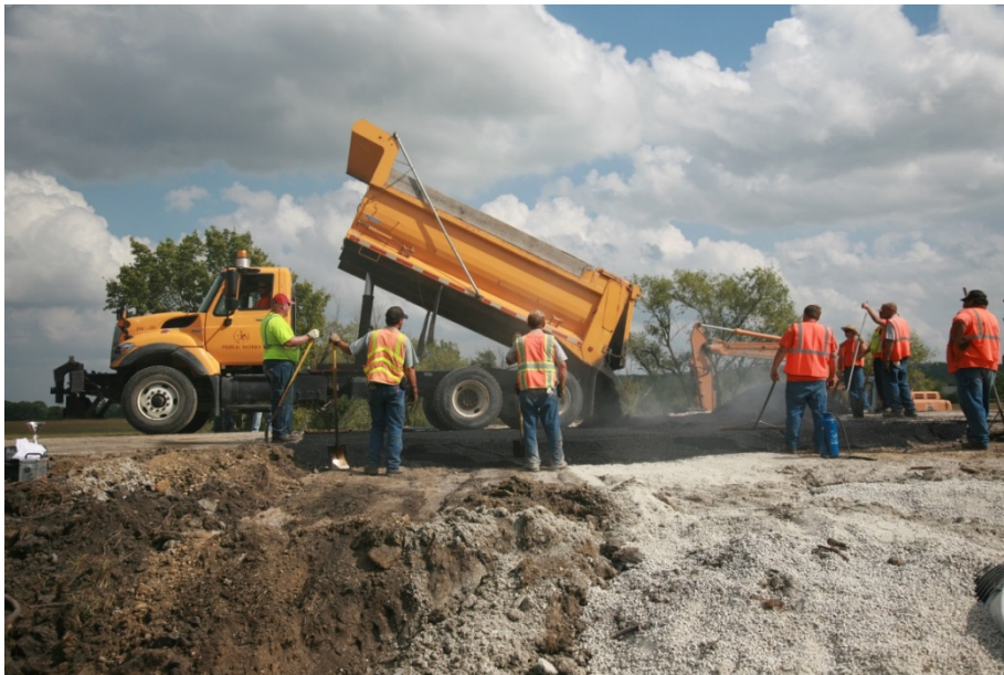
FIGURE 5.26 A truck dumping HMA for the HMA surface
