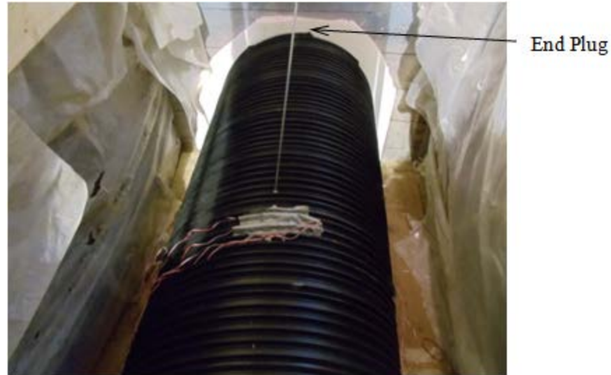
FIGURE 4.17 Fully instrumented pipes in the trench in Test Section 1
