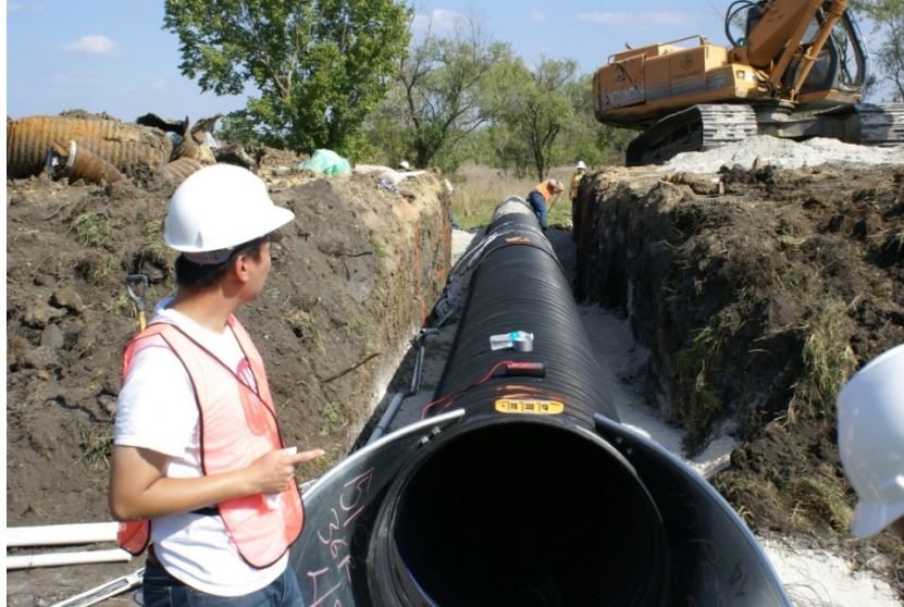
FIGURE 5.17 Fully instrumented pipes in the trench
