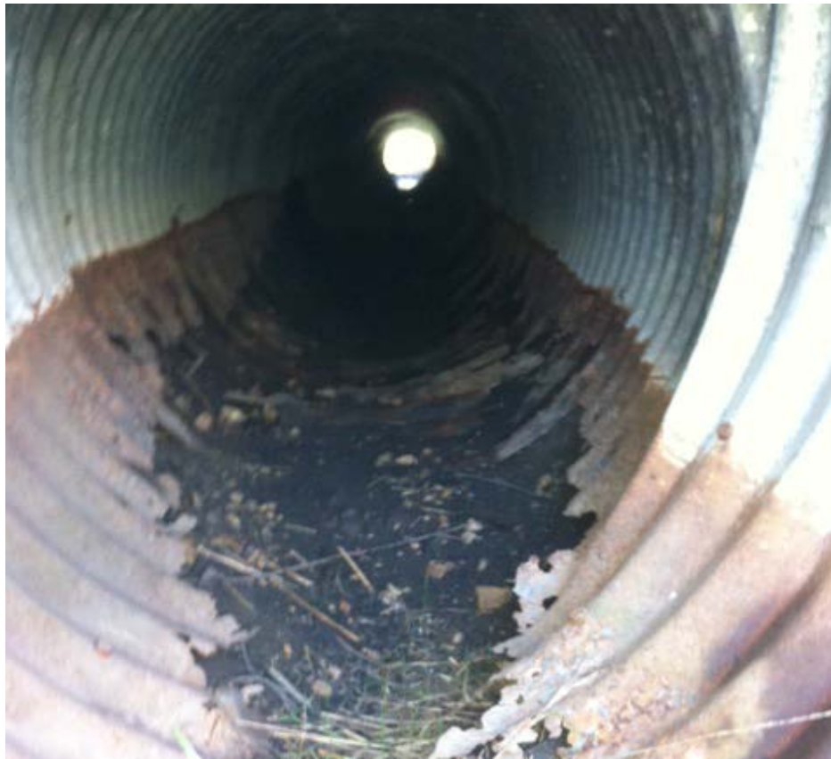
FIGURE 5.9 An existing corrugated metal pipe under service
