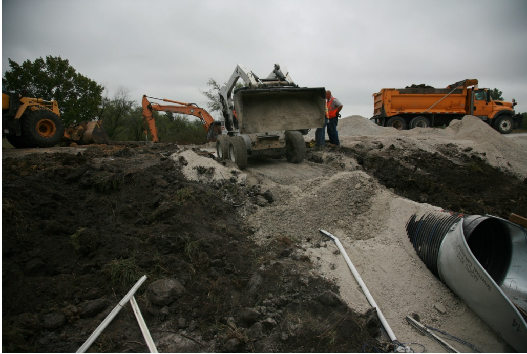
FIGURE 5.20 A bobcat used to dump and level soils
