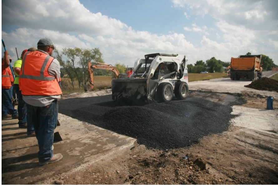
FIGURE 5.27 HMA dumped and leveled using the bobcat
