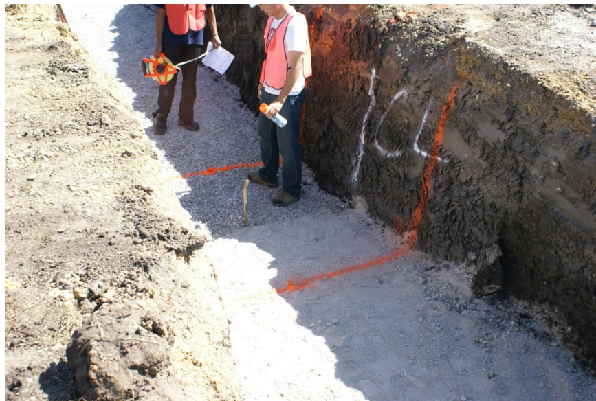
FIGURE 5.13 Marking wheel paths
