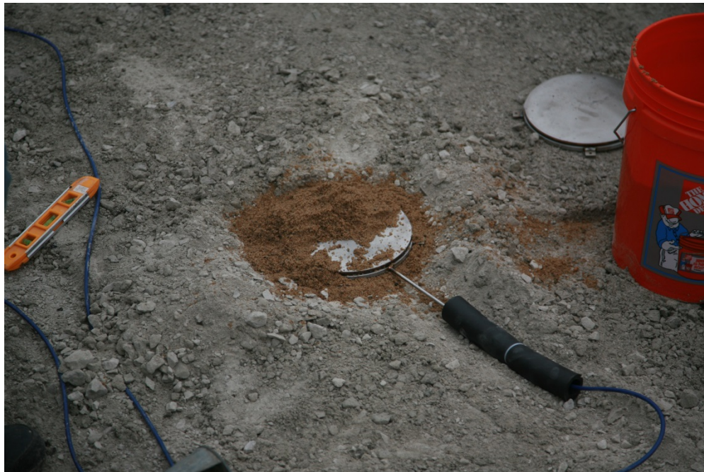
(b) At pipe crown
