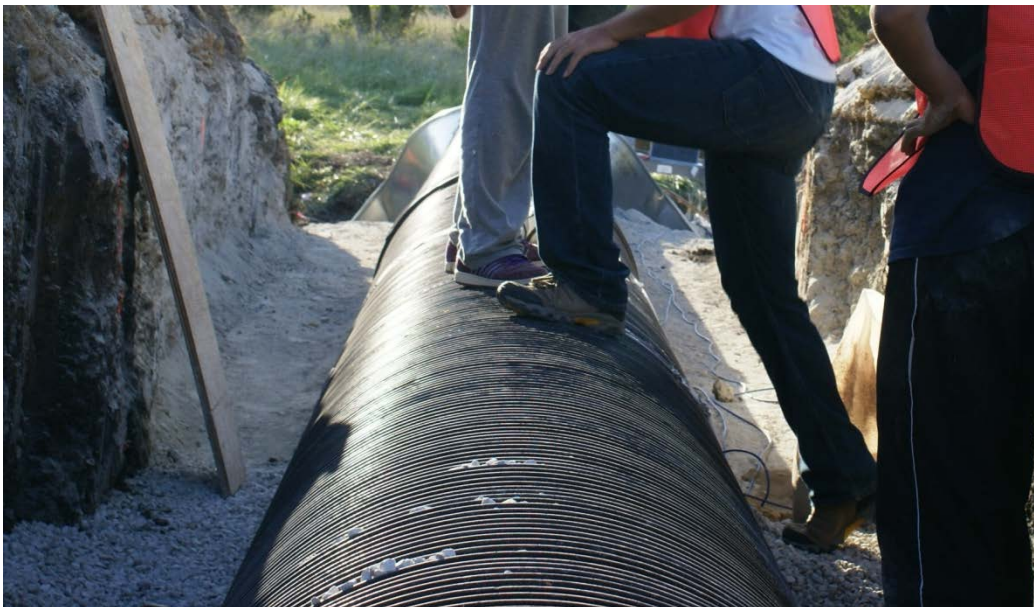
FIGURE 5.19 Backfilling up to springline
