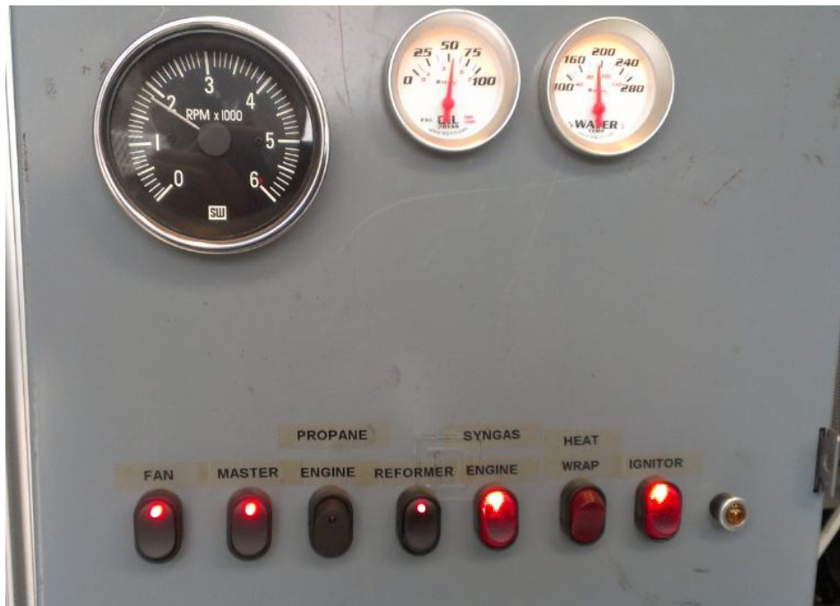
Figure 32 - Control panel during reformed propane combustion
