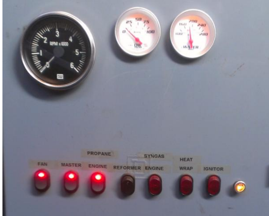
Figure 25 - Syngas control panel for engine combustion using pure propane
