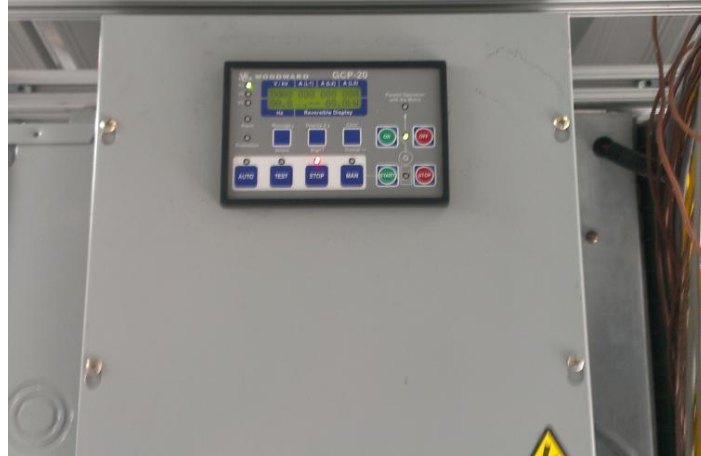
Figure 12 - GCP 20 generator controller
