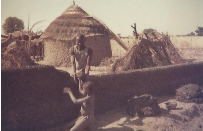
Figure 36: The Beginning of the Change; a Man and Son Building Mud Wall Fence
