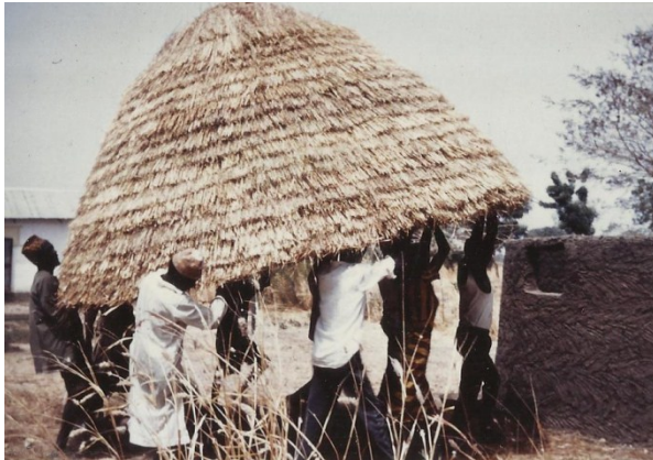
Figure 34: Finished Roof Being Raised, to be placed on Top of the Mud Hut
