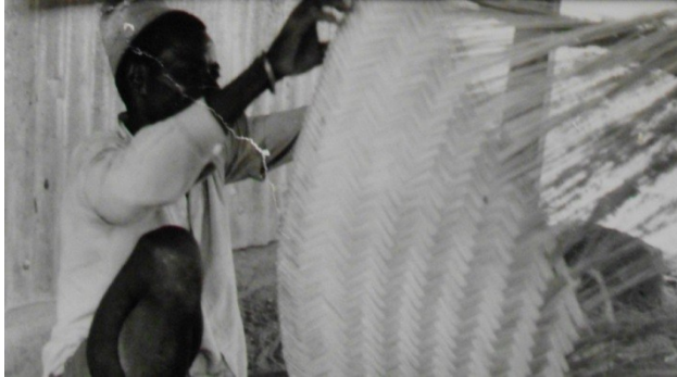
Figure 33: The Roof Cap-Like Top Cover ( Wata ) being woven
