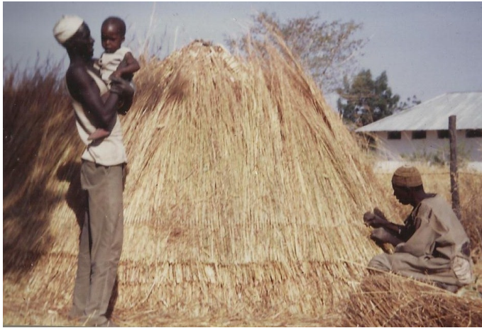
Figure 32: Roofing; the Roof Structural Frame being covered with Misham
