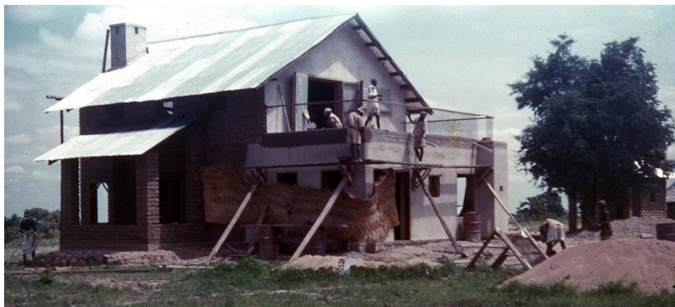
Figure 57: The Residence under Construction
