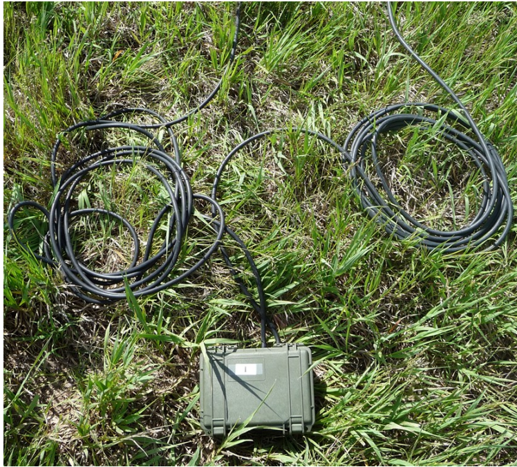
Figure 4.10 A Speed Measurement Sensor Connected with Road Tubes
