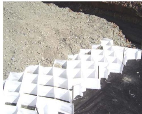
Figure 2.7 Placement of soil in geocell
