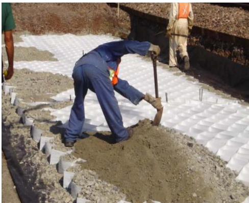
Figure 2.6 Placement of soil in geocell
