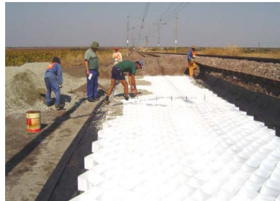
Figure 2.5 Placing geocell
