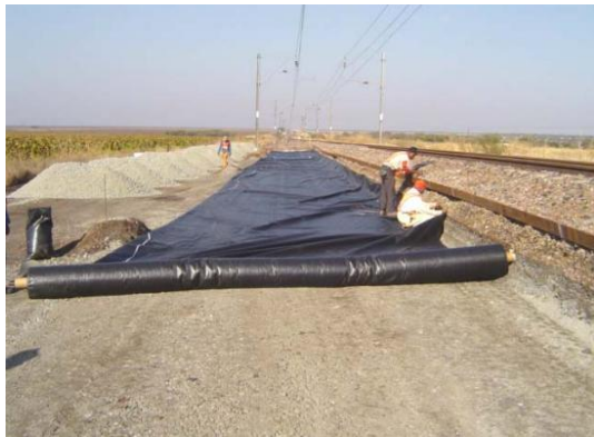
Figure 2.4 Placing geotextile sheet
