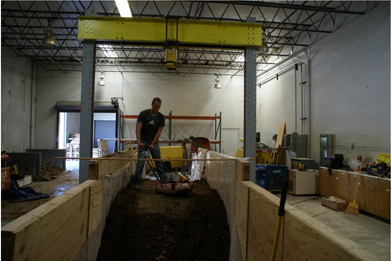
Figure 3.11 Placing subgrade and compaction
