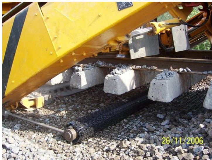
Figure 1.3 Placement geogrid under railroad track
