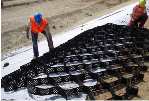
Figure 1.1 Placing geocell in the field
