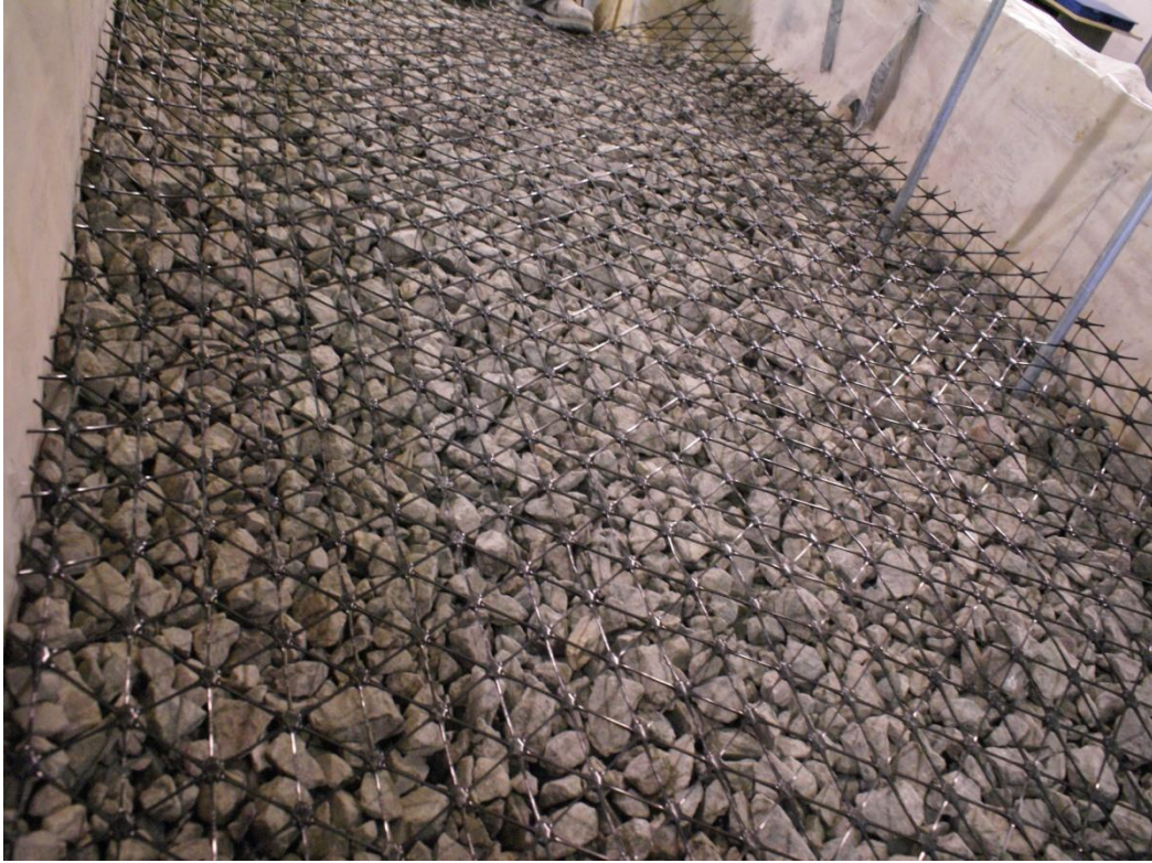
Figure 4.2 Geogrid after replacement in the reinforced test
