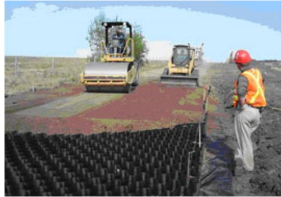
Figure 1.2 Filling geocell
