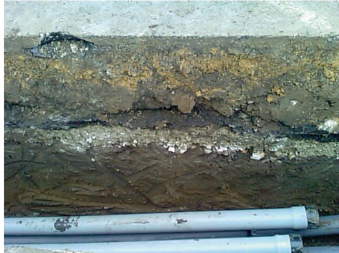
Figure 10. Layers of urban land use are apparent in this trench on the University of Kansas campus in Lawrence, KS. Pipes shown are approximately four inches in diameter. Photograph by T. Jackson.
