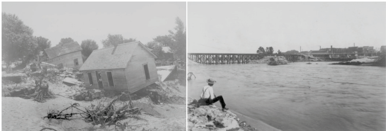
Figure 25. The flood of 1903 caused extensive damage to infrastructure along the Kansas River, including the Bowersock Dam. Many houses in North Lawrence were flooded, and some were swept away (left). In the right image (looking southeast), an onlooker watches debris pile up against the Massachusetts Street bridge, which eventually led to the destruction on its northern span (USGS 1903, Kansas Water Science Center 2009).
