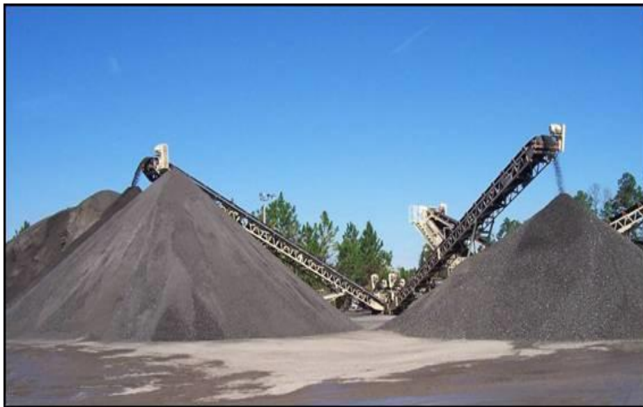
Figure 2.2.1 Processing and stockpiling of RAP ( http://www.fhwa.dot.gov/PAVEMENT/recycling/rap/index.cfm )
