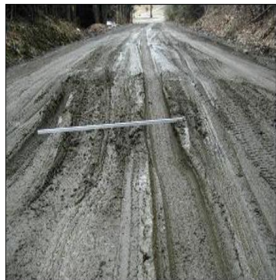
Figure 1.2.2 Rutting in unpaved road (Courtesy of Dr. Han)
