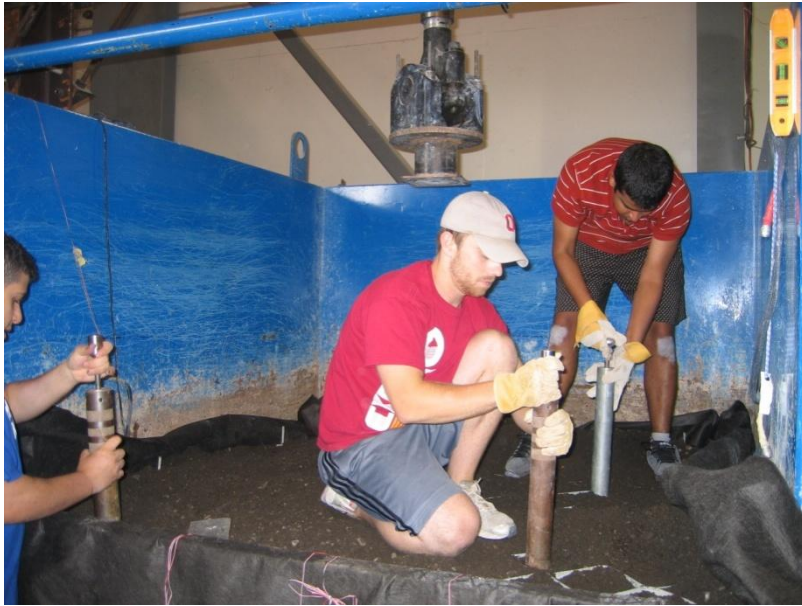
Figure 5.2.5 Compacting RAP inside the geocell by hand tamping
