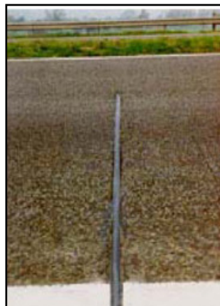
Figure 3 Piezoelectric Sensor (8)
