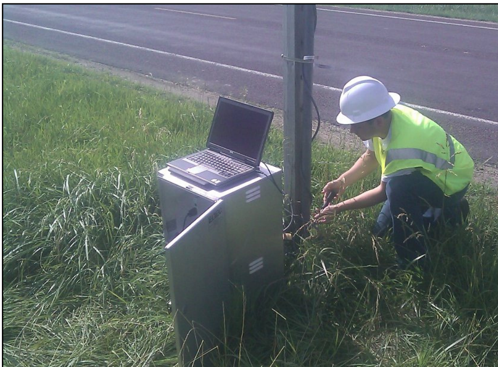
Figure 27 Smartsensor Setup
