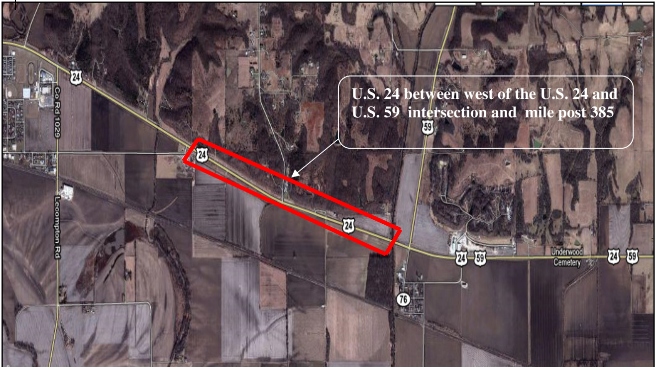
Figure 18 U.S. 24 Between West of U.S. 24 and U.S.59 Intersection and Mile Post 385
