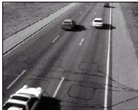
Figure 1 Inductive Loop Detector System (7)
