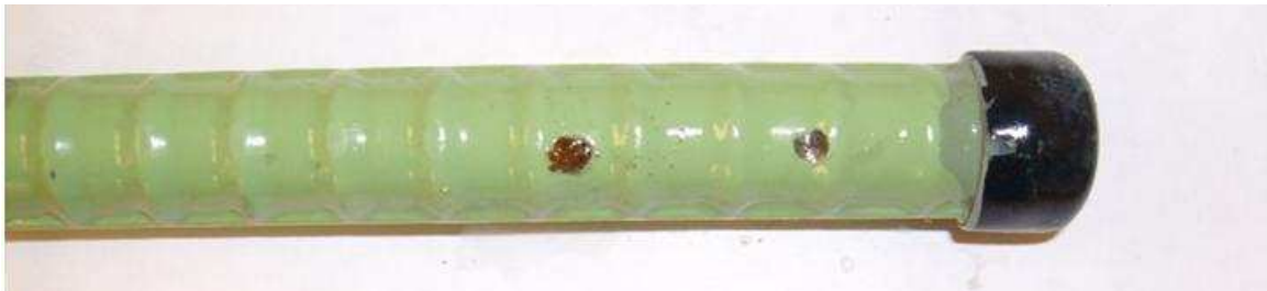
Figure 3.95: Rapid macrocell test, M-ECR-1, 5 weeks, before disbondment test.
