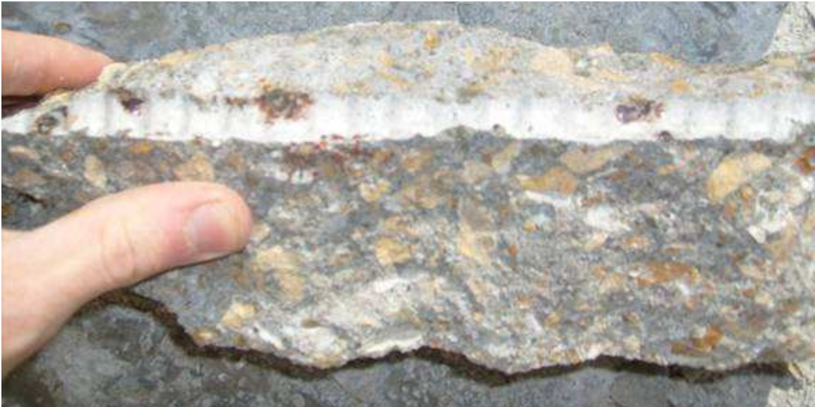
Figure 4.24: Concrete surrounding test bar from specimen 2h-V-1.
