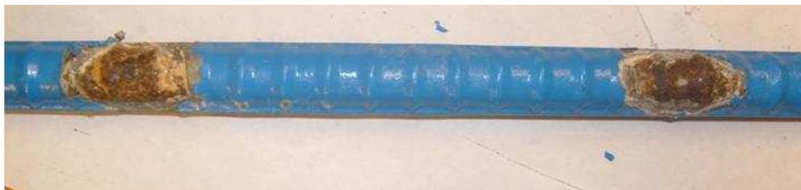
Figure 3.87: FTS-ECR(RH)-C-1, showing severe disbondment on a bar from the top mat of steel.
