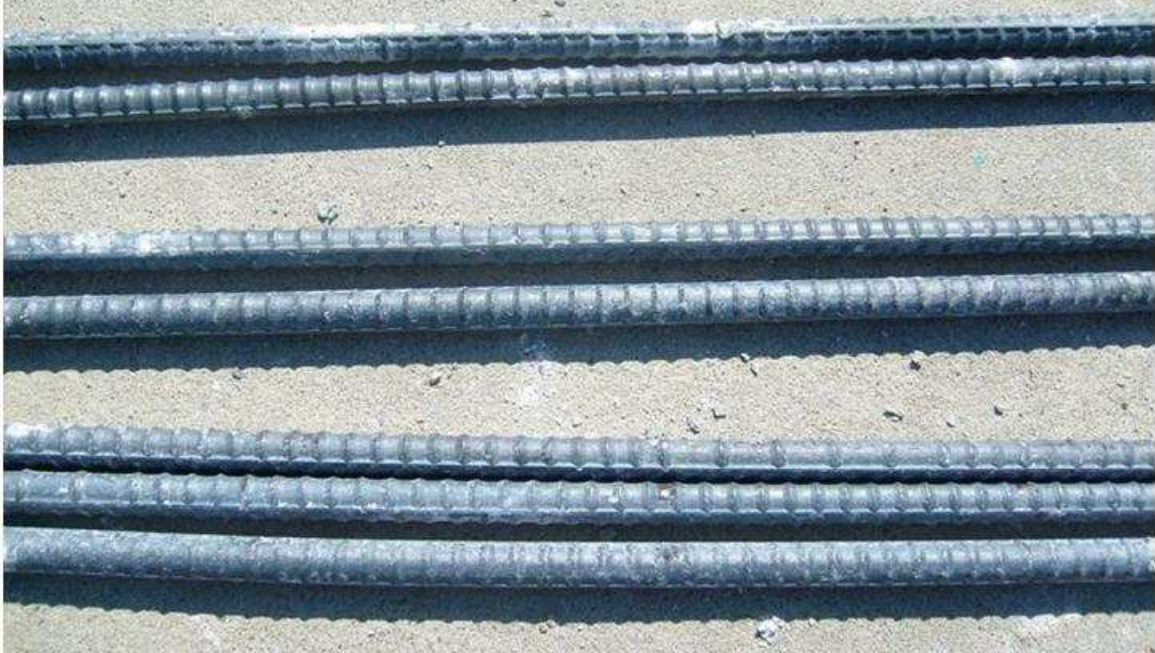
Figure 3.71: Specimen FTS-Conv.-U-2, bottom mat of steel.
