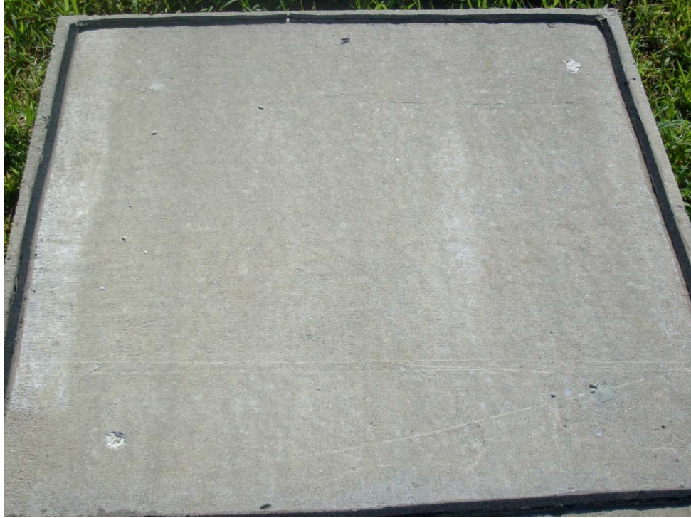
Figure 3.66: Specimen FTS-ECR-U-2 at end of test.
