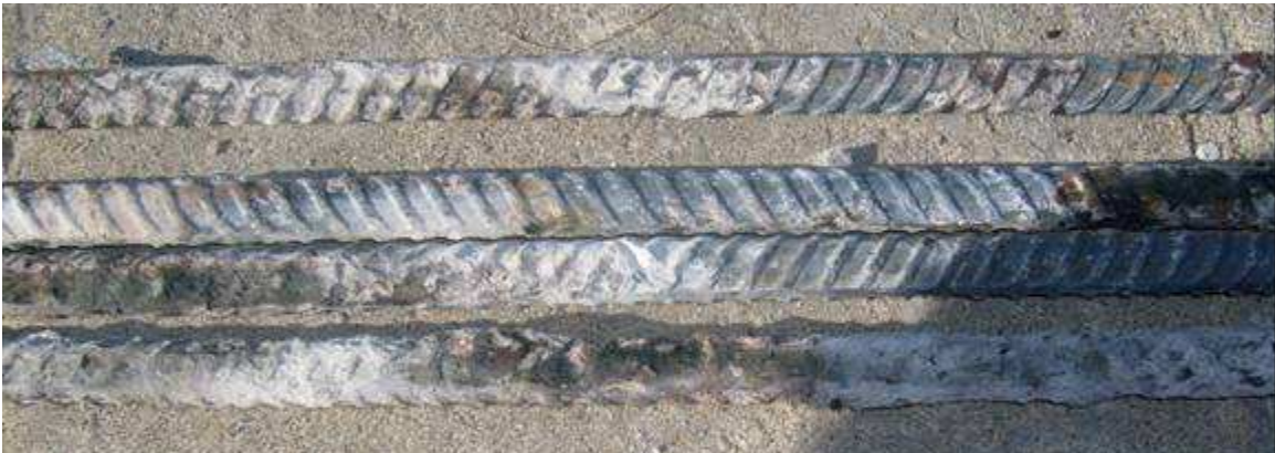
Figure 3.144: Specimen FTS-DCB(Conv.)-1, selected bars from top mat of steel showing heavy corrosion.
