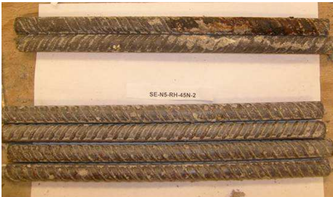
Figure 3.9: Specimen SE-Conv.2-RH-2, 96 weeks. Steel in top mat (above label) and bottom mat (below label).
