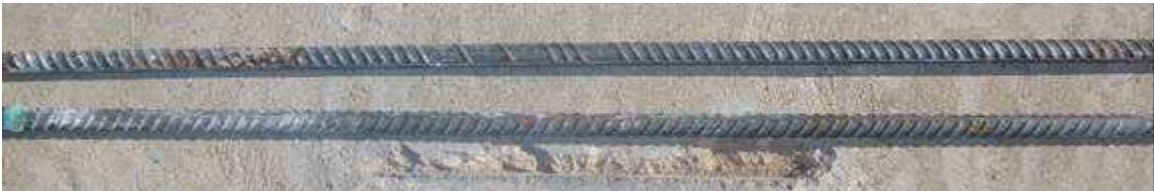
Figure 3.145: Specimen FTS-DCB(Conv.)-1, selected bars from bottom mat of steel showing moderate corrosion.
