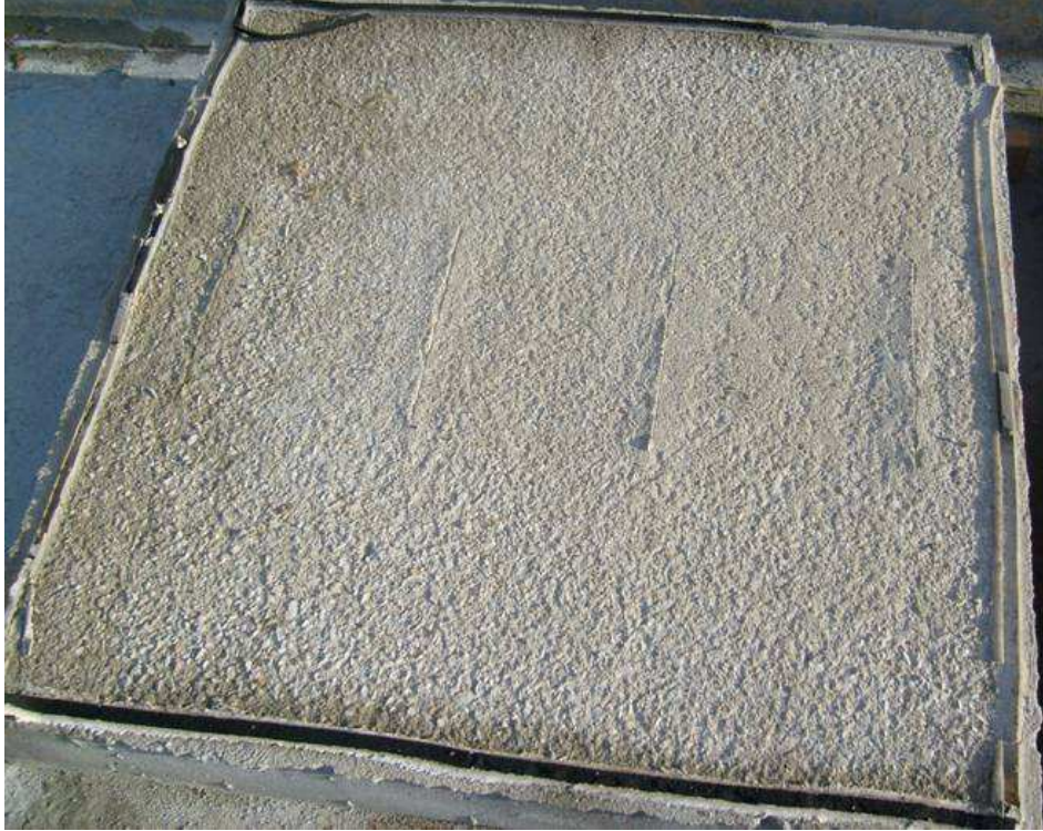
Figure 3.68: Scaling on specimen FTS-ECR(HY)-C-2 at end of test.
