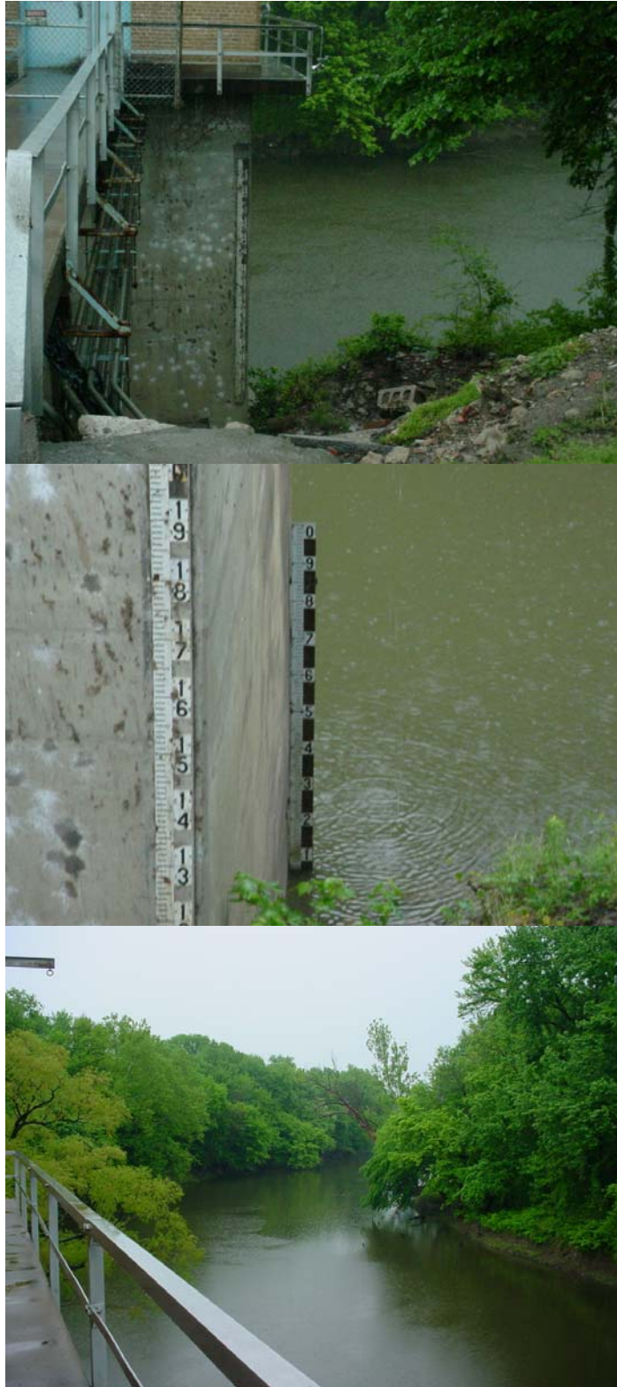
Figure 3-4. NWS staff gage at Coffeyville- three views. http://www.crh.noaa.gov/ahps2/hydrograph.php?wfo=ict&gage=cfvk1
