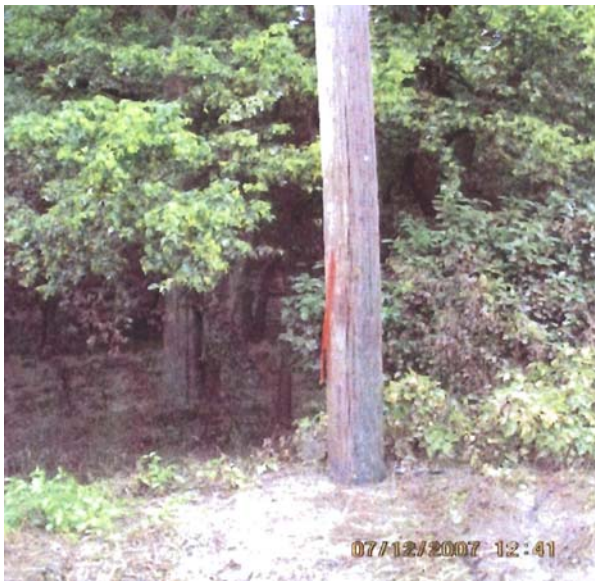
Figure 3-8. HWM in situ photos. Two examples of locations from which high water marks were surveyed after the 2007 flood, one on the side of a home and the other on a utility pole (USACE, 2007).
