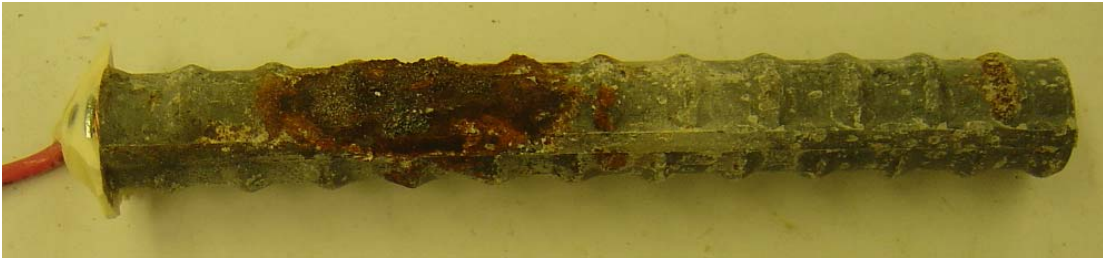
Figure 3.15 – Macrocell Test. Conventional steel from anode specimen (M-Conv.-HY45-1) showing severe corrosion products at week 15.
