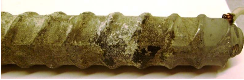
Figure 3.138 – Initiation Beam Test. Zinc-coated reinforcement after autopsy (B-Zn-45N-4) showing corrosion on the bottom bar exposing underlying steel.
