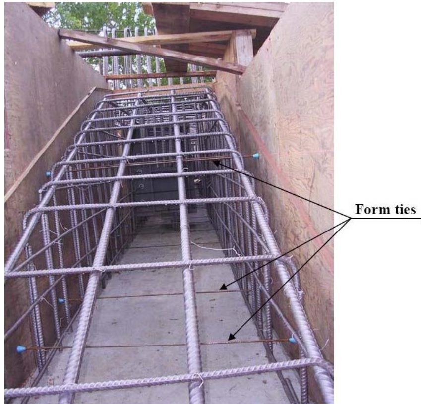
Figure 3.116 – Reinforcing bar cages at the east abutment for the Mission Creek Bridge, showing mild steel form ties used in the bridge decks.
