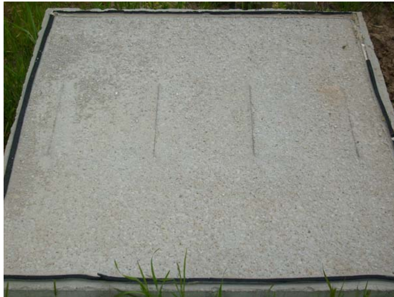
Figure 3.92 – Field test specimen ECR(Hycrete) (2) with simulated cracks at week 169, showing scaling on the surface.
