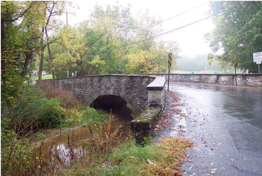
Figure 2.9 An old stone arch bridge in Pennsylvania (Source: PENNDOT, 2008)
