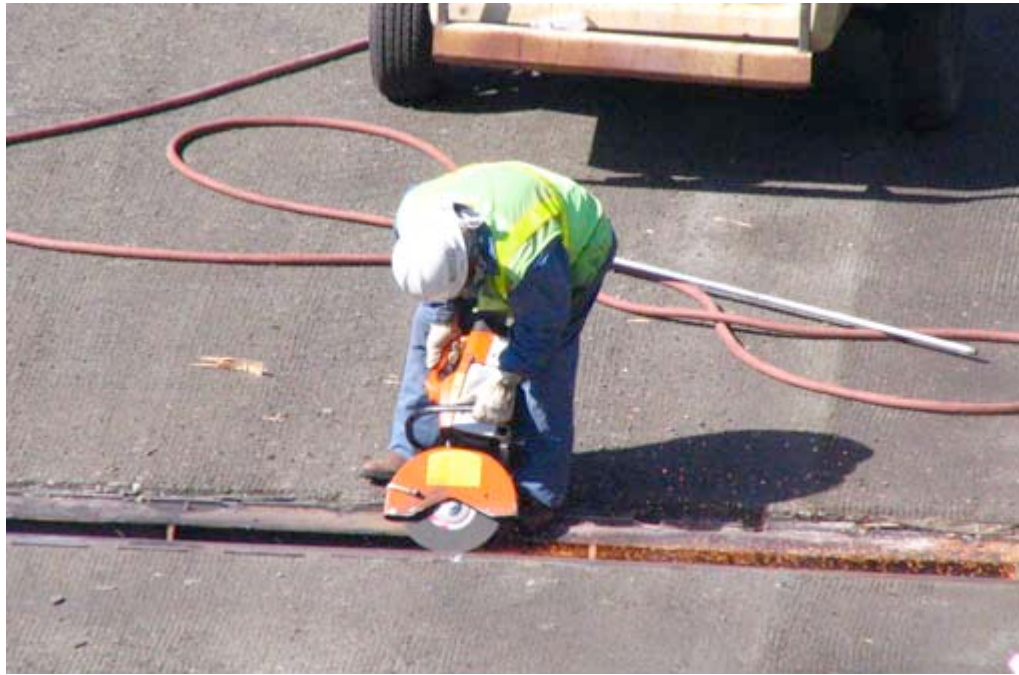
Figure 4.7 A Sample Bridge Expansion Joint During Maintenance (Source: WSDOT, 2009)
