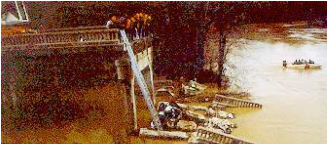
Figure 2.2 Hatchie River bridge (Source: Turne- Fairbank Highway Research Center, 1995)
