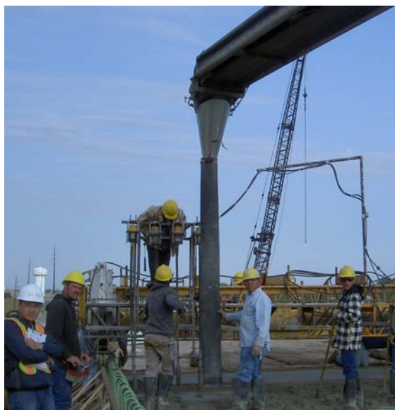
Fig. 5.14 – Typical conveyor drop for LC-HPC-11
