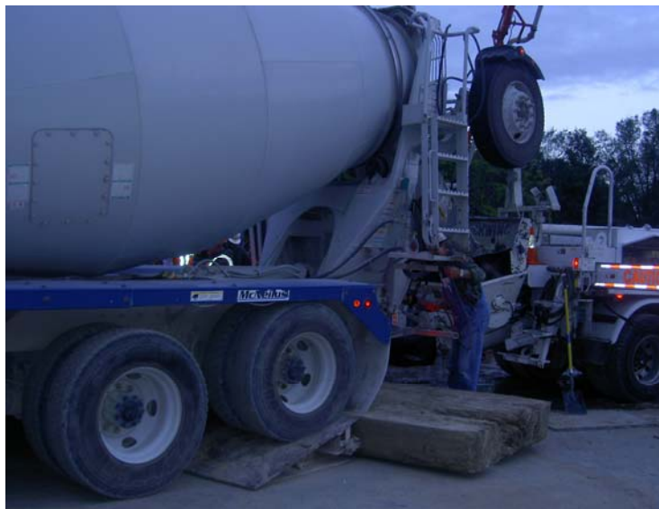
Fig. 5.4 – Example of a ramp used by ready-mix trucks to increase the chute angle and facilitate unloading the relatively low-slump LC-HPC.
