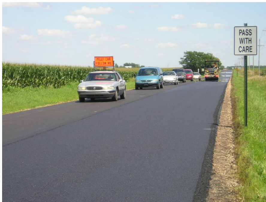
Figure 24. Traffic control (single lane closure)
