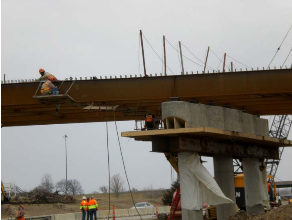
Figure 45. Bolting Operation on the Edge Span
