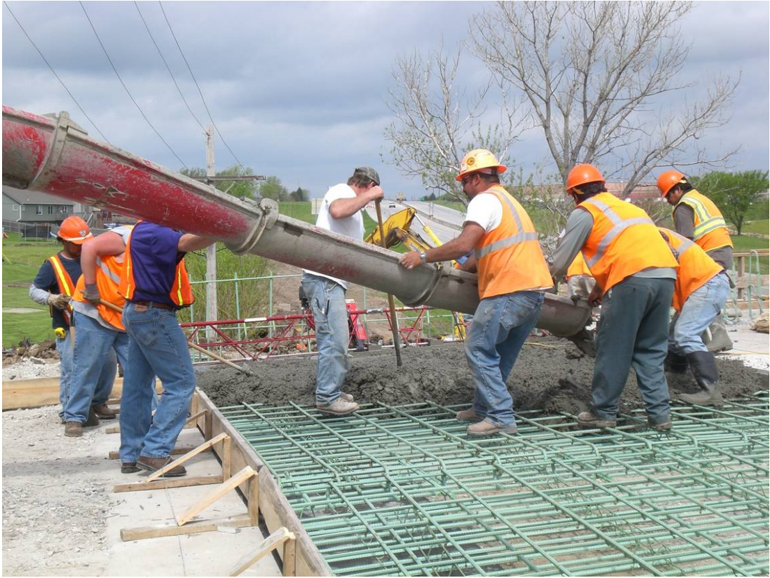
Approach Road Pouring
