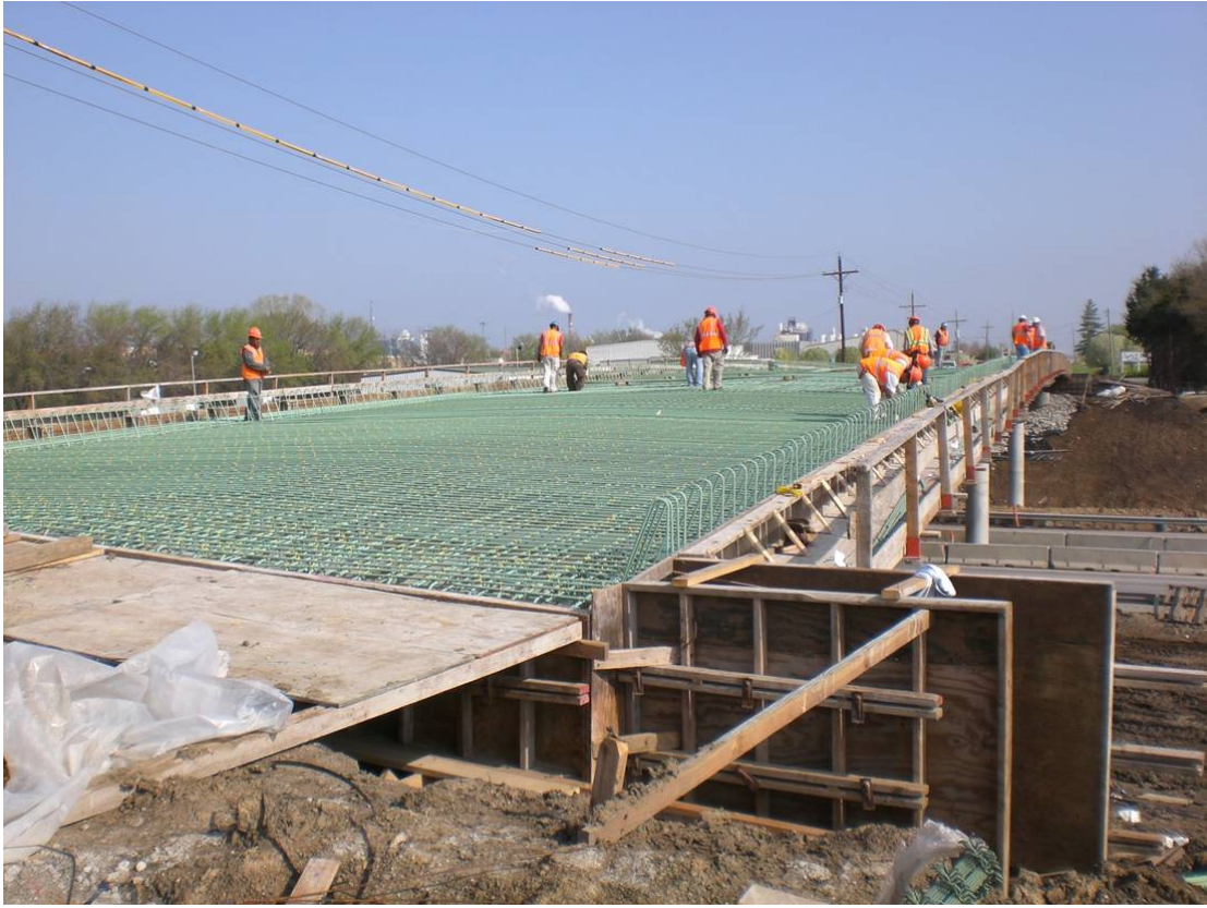
Placing Rebar
