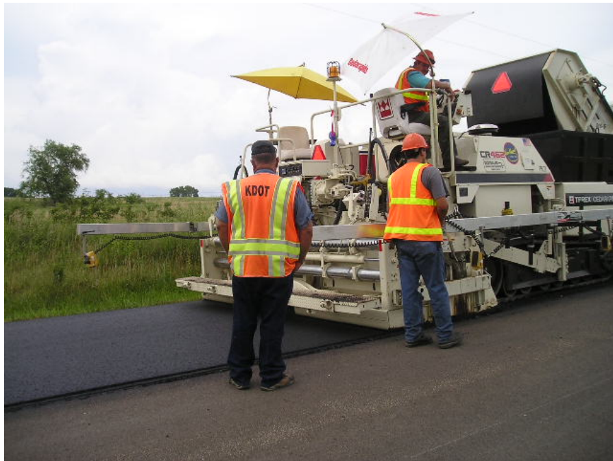
Figure 35. Surface paving equipment
