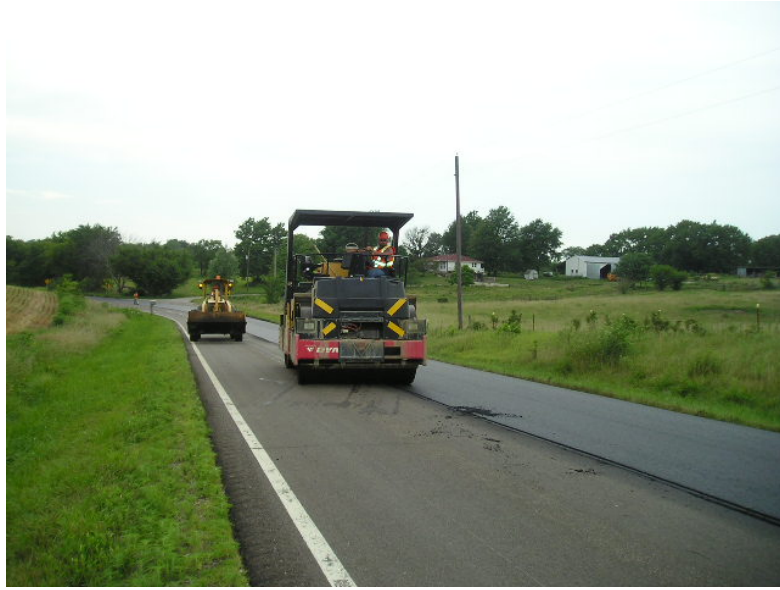
Figure 36. Compaction
