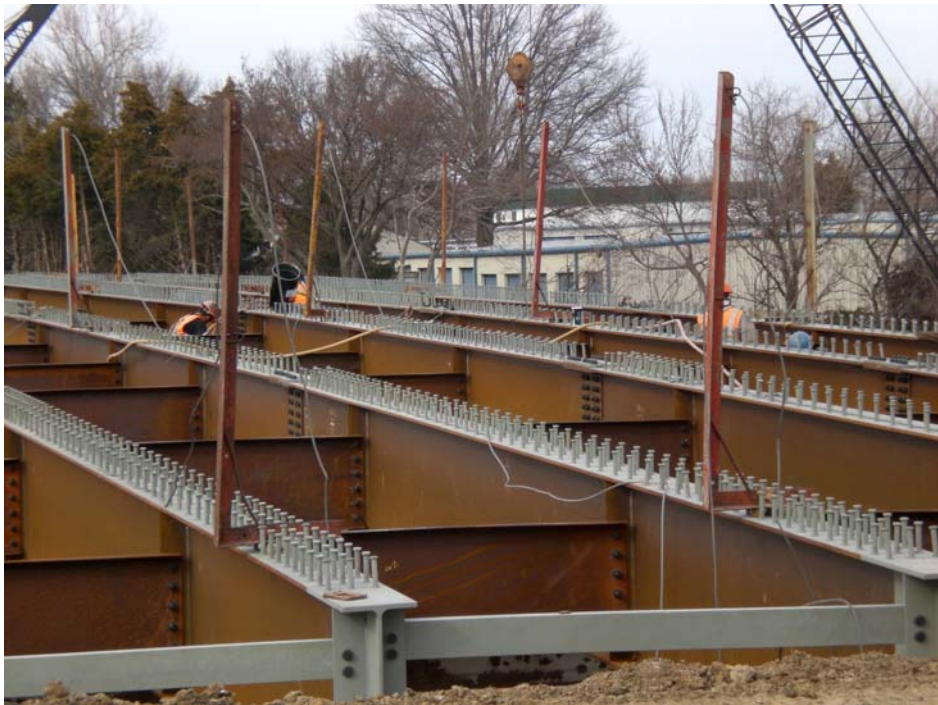
Figure 46. Bolting Operation on the Middle Span
