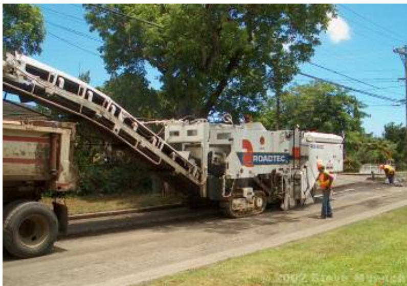
Figure 25. Milling (Washington Asphalt Pavement Association 2002)
