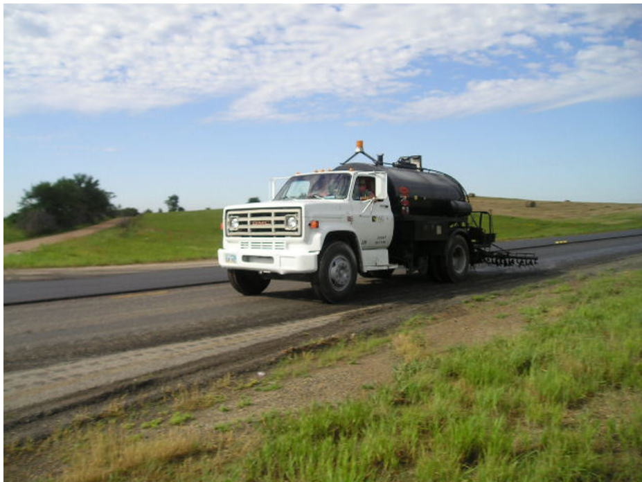
Figure 26. Tack coat material applied by a pressure distributor
