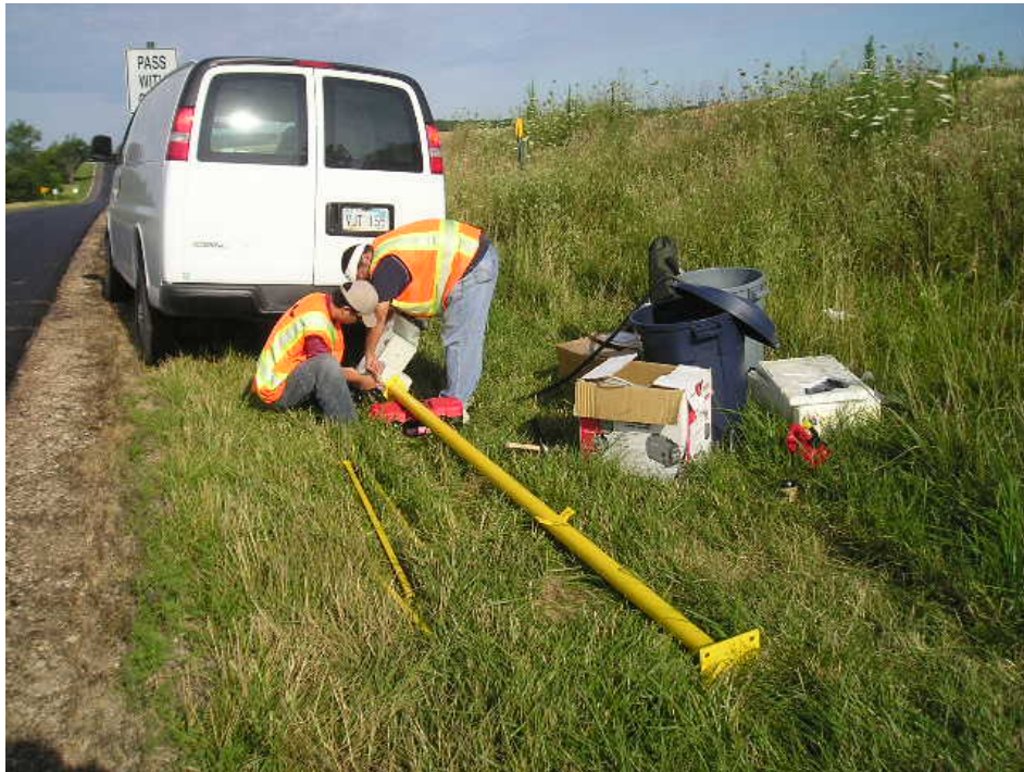
Figure 15. Mounting camera on the pole
