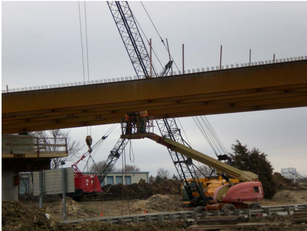
Figure 47. Bolting Operation using Jumbo Lift
