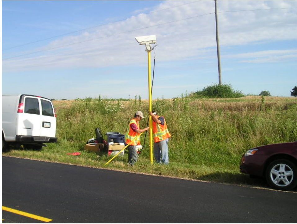
Figure 17. Supporting the pole with three steel legs
