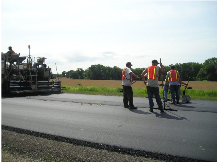
Figure 28. Sampling the asphalt mix for lab test
