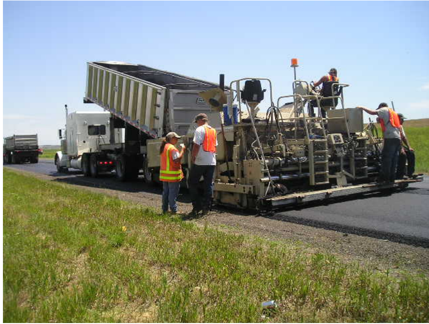
Figure 27. HMA paving
