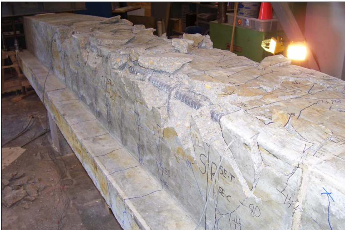
Figure B.39 – Specimen 11-8-XC2-2 at the conclusion of the test
