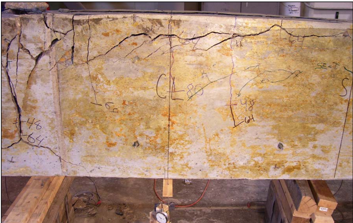
Figure B.28 – Specimen 11-8-OC0-2 at the conclusion of the test
