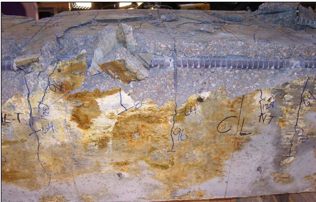
Figure B.37 – Specimen 11-8-XC1-2 at the conclusion of the test
