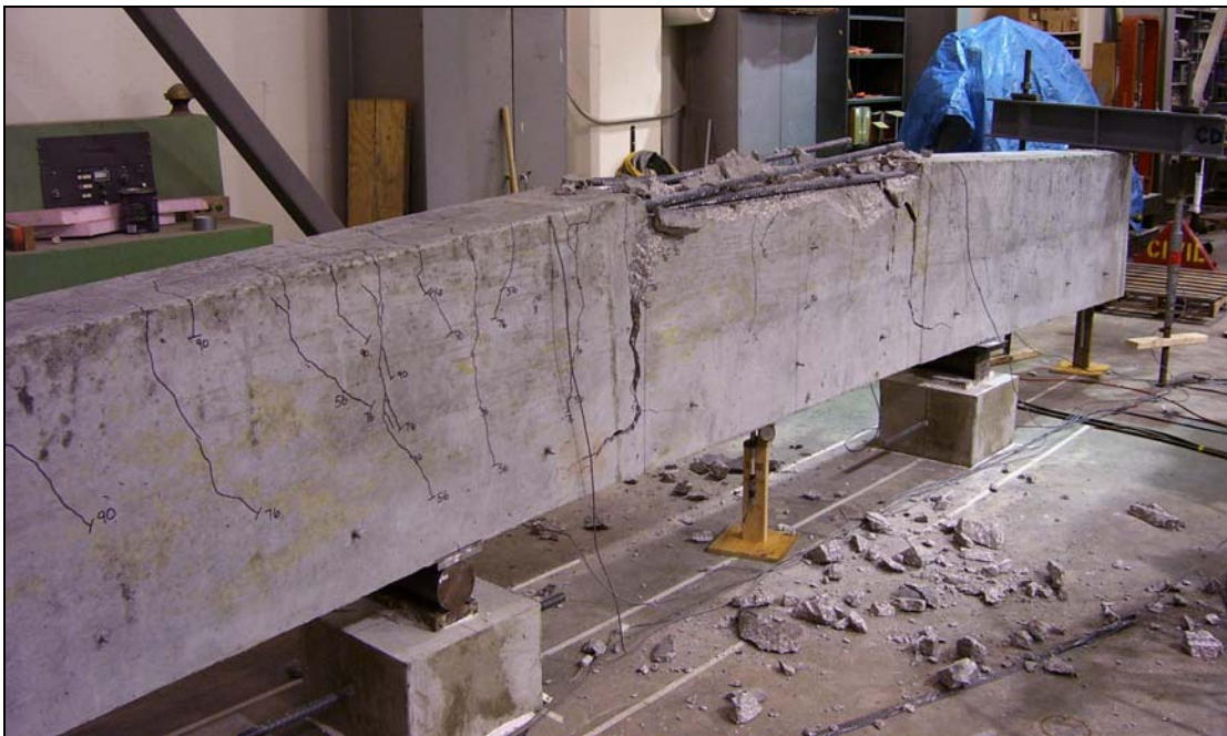
Figure B.13 – Specimen 8-5-XC0-1.5 at the conclusion of the test
