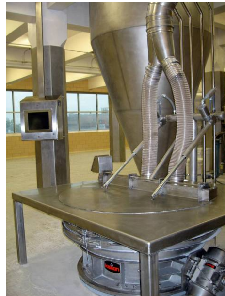
Exhibit 10: Hopper and Dump Station Installed
