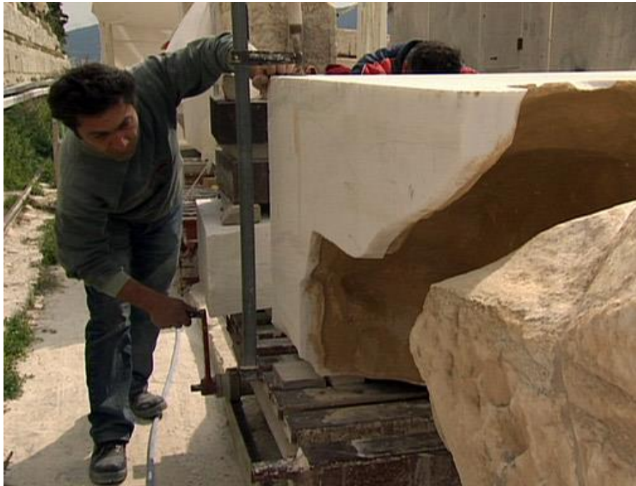
Figure 5.1 Mating of two marble blocks [193].
