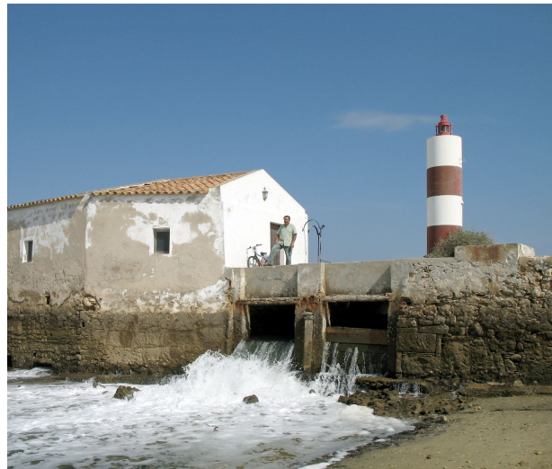
Figure 3.4: A Medieval Tide Mill in Olhao Portugal Notice the sluice gates controlling the flow of water [7].
