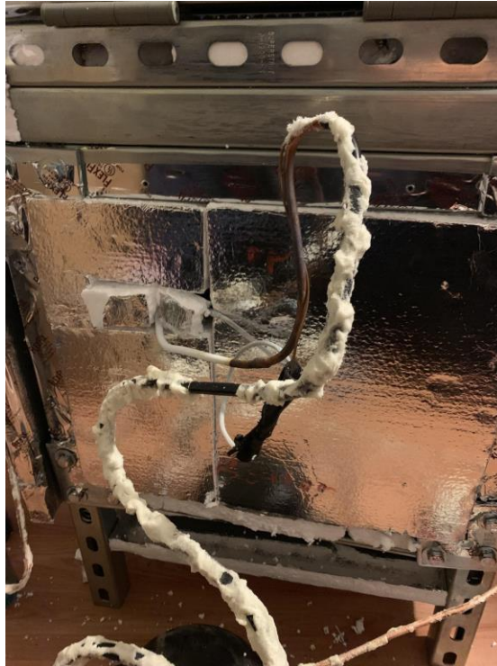
Figure A.6: The compressor unit being fitted on and installed into the unit.
