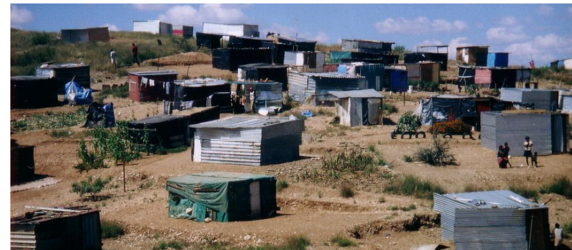
Figure 4: Informal Settlement, Katutura (Nyangove, 2010)
