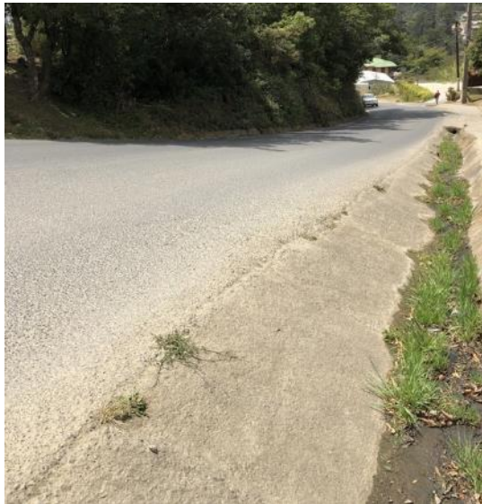
Figure 18: Drainage ditch on the side of a road
