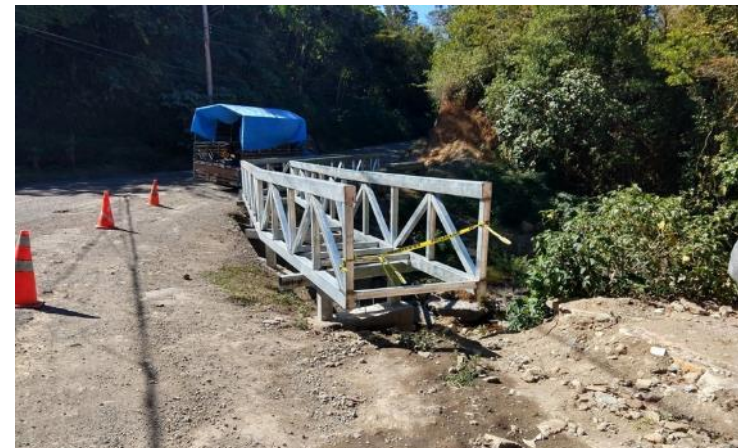
Figure 21: Bridge under construction in Monteverde
