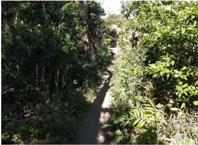
Figure 17: Overgrown pedestrian path
