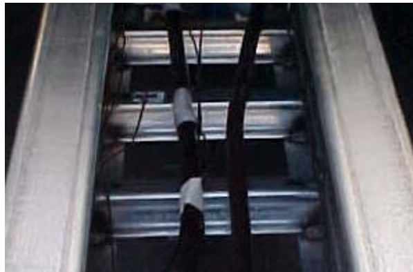
Figure 3-1 Single Cable Experiment in Cable Tray
