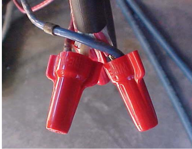
Figure 3-10 Wire Nut Connections
