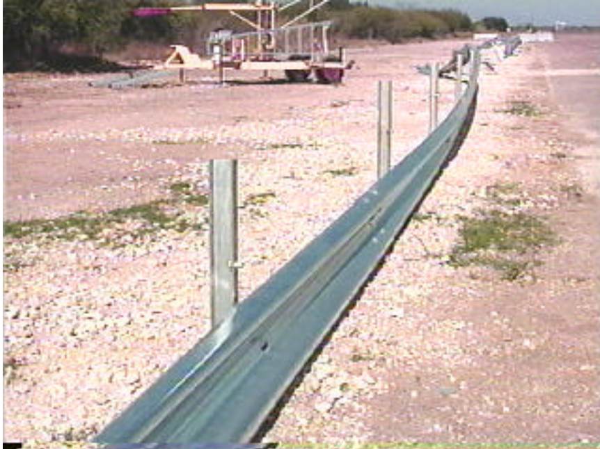
Figure 54: Damage looking up-stream from the impact point.
