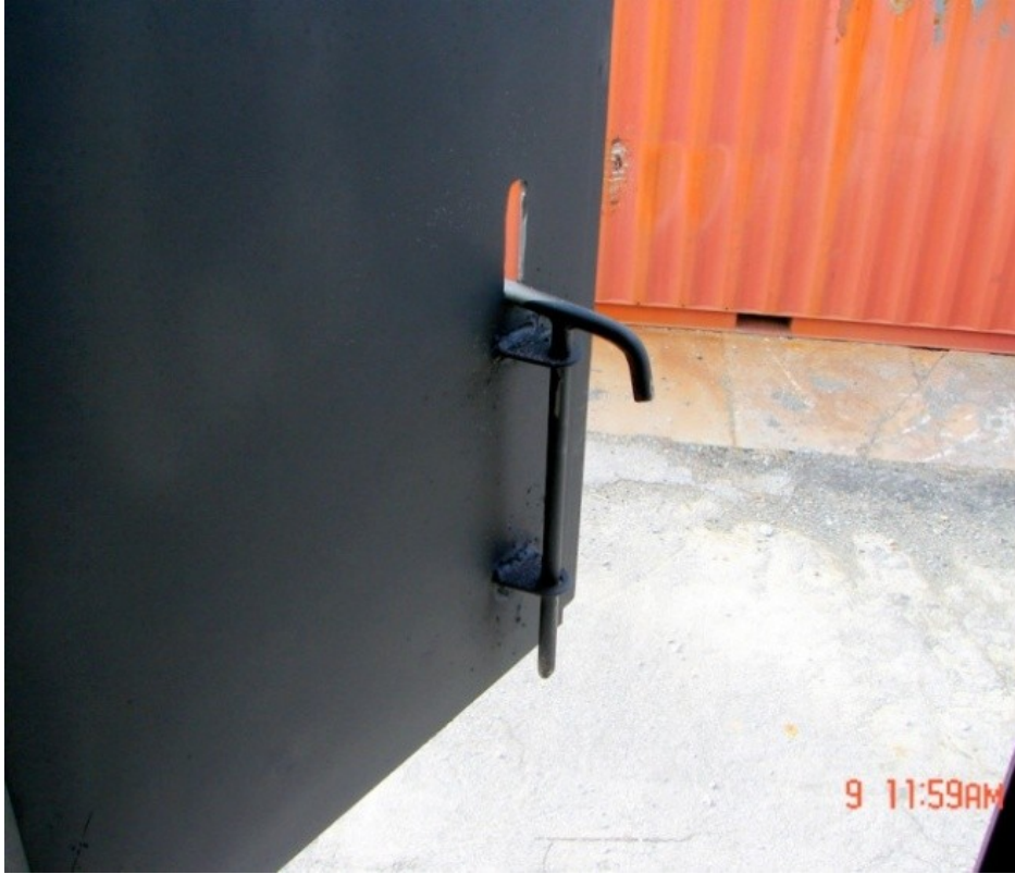
Figure 4-11: Window & Latch Construction
