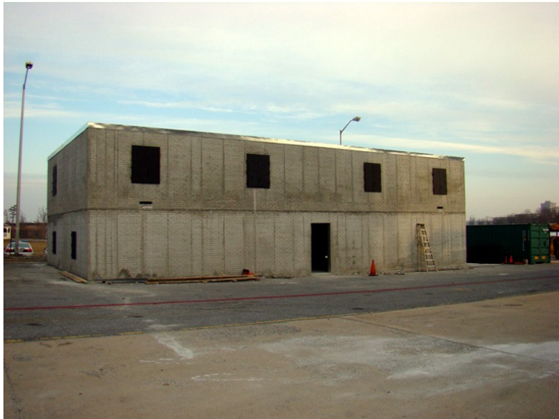
Figure 4-5: View of A-B corner of the burn facility
