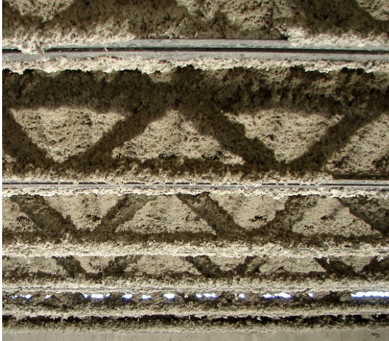
Figure 4-9: Fireproofing added to structural steel
