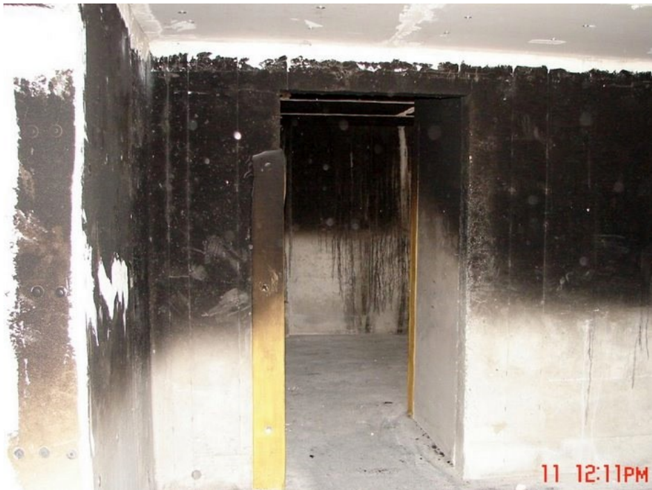
Figure 4-12: Interior view of Burn Facility
