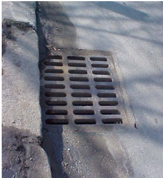
Figure 20: Example of Roadside Drainage
