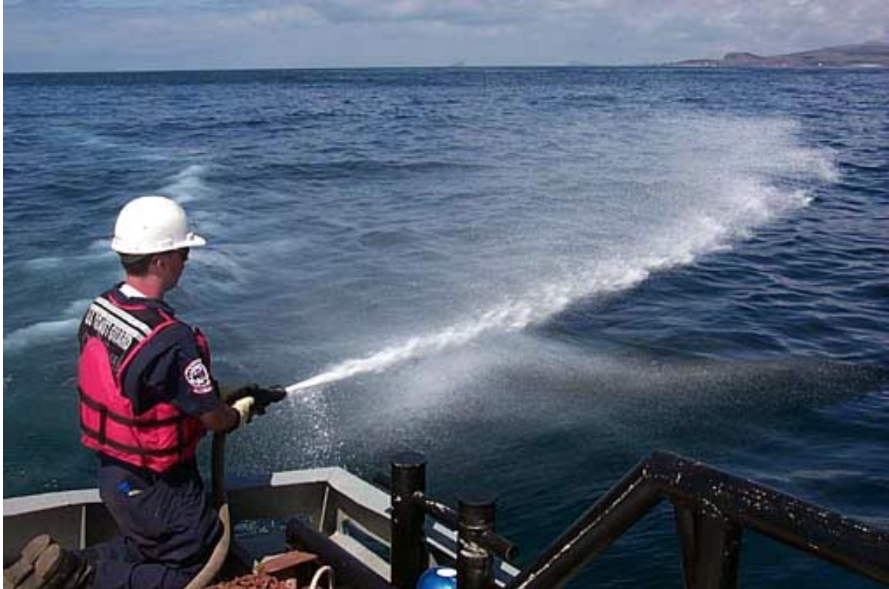
Figure 6: Oil spill clean-up using chemical dispersants [20]
