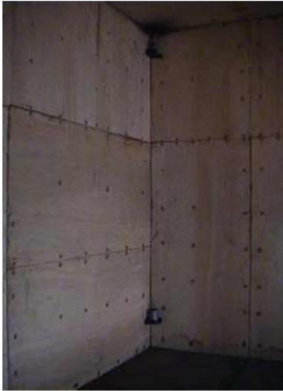
Photograph 5. Inside of Enclosure
