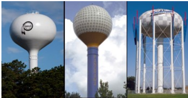
Figure 3.1 Left: Spheroid, Middle: Pedesphere, right: Multicolumn sphere [74]
