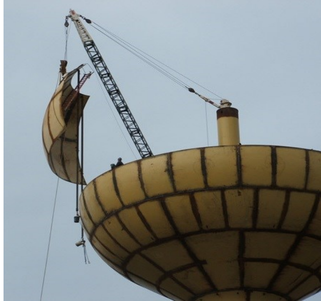
Figure 3.3 Construction of large elevated spherical tank
