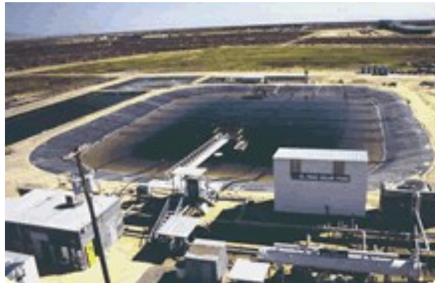
Figure 2.2 Solar pond in El Paso Texas [47]
