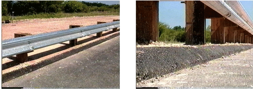
Figure 2.10: Guardrail/curb installation for TTI test 404201-1.(32)
