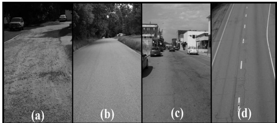
Figure 19. Images of local road surface characterization including (a) unpaved roads, (b) paved secondary roads, (c) paved city streets and, (d) paved multi-lane highways
