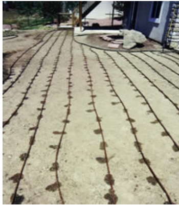
Photograph 6: A small scale drip irrigation system ( http://www.xeriscape.net/images/SubIrrigationSite.jpg )
