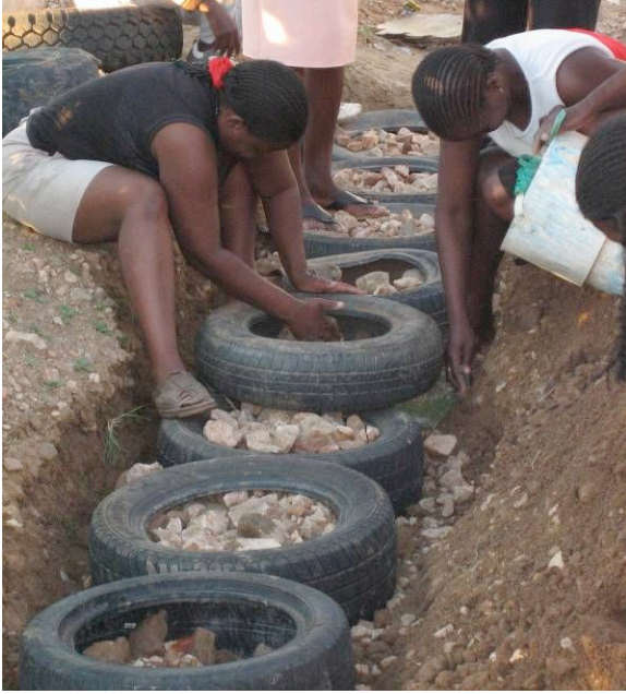
Figure 11: Site #3 During Construction
