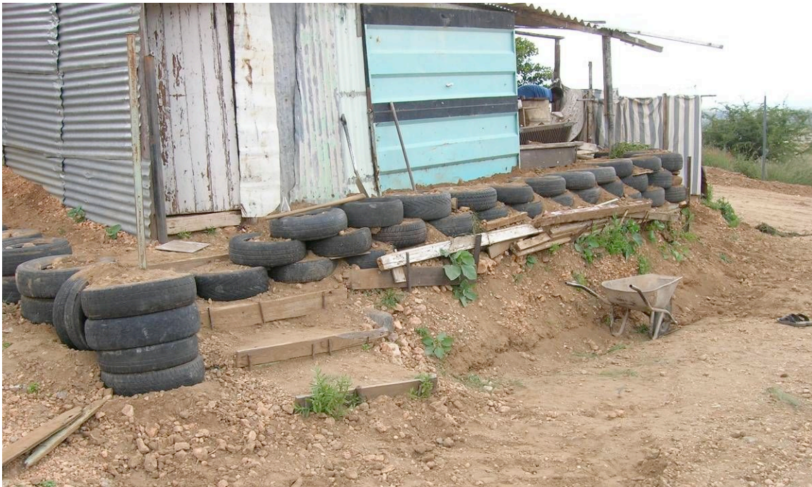
Figure 16: Tyre Reinforcement of the Embankment Around Joseph's House
