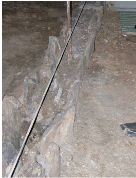
Figure 17: Independently Developed Wall of Concrete and Stones
