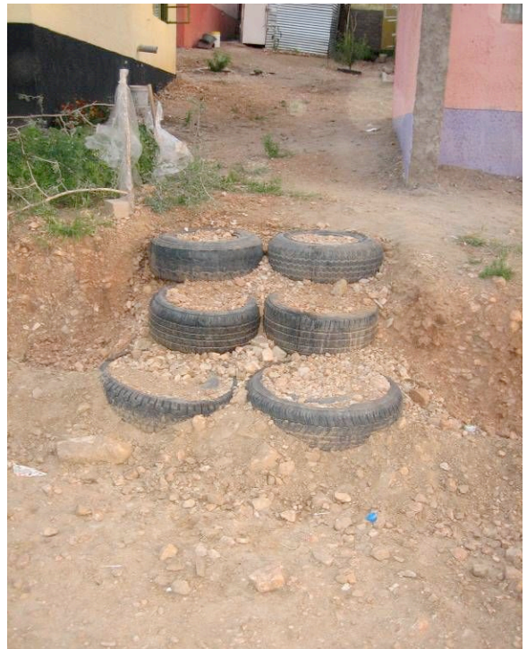
Figure 14: Completed Tyre Steps at Site #4
