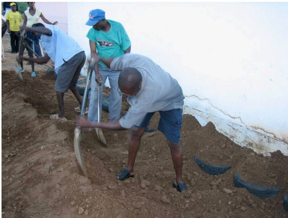
Figure 8: Construction of a Tyre Wall at Site #1
