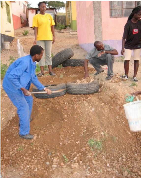
Figure 13: Construction of Tyre Steps at Site #4
