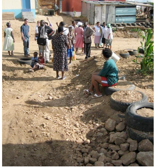
Figure 12: Finished Tyre Wall at Site #3
