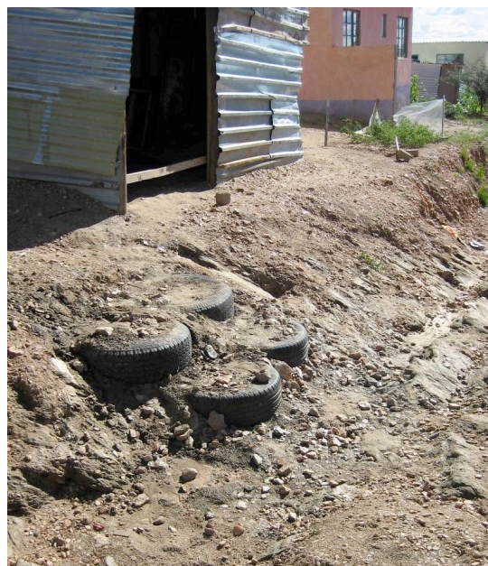
Figure 15: Independently Developed Tyre Steps
