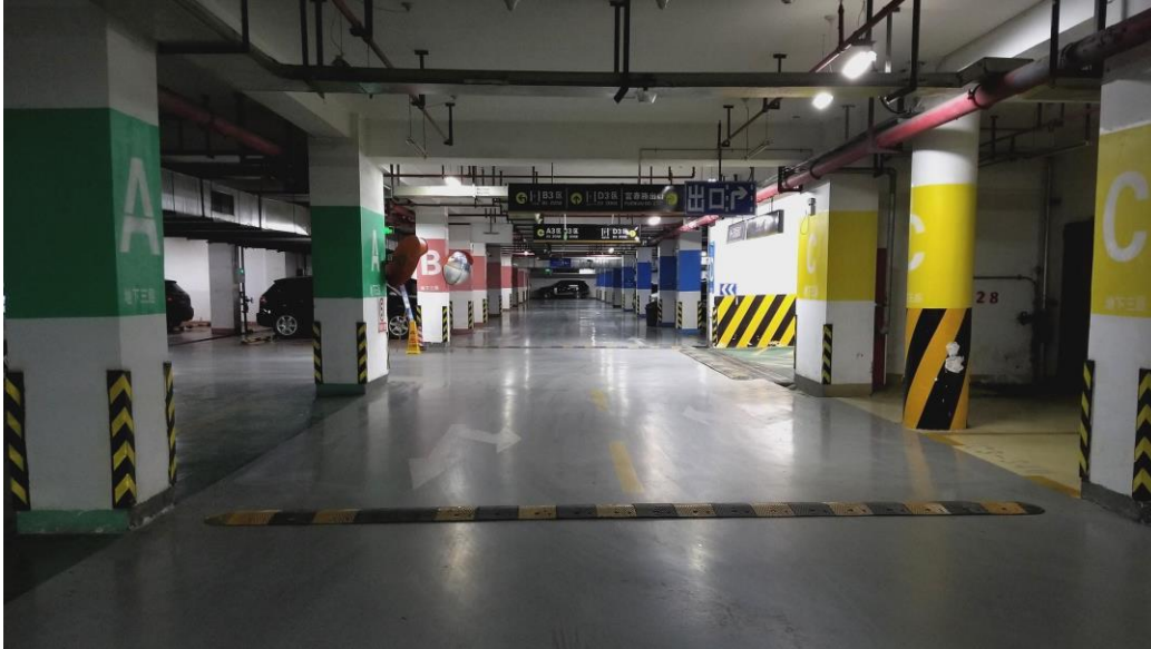
Figure 16: Parking complex floor divided into sections by colors and letters, Qianjiang New Town
