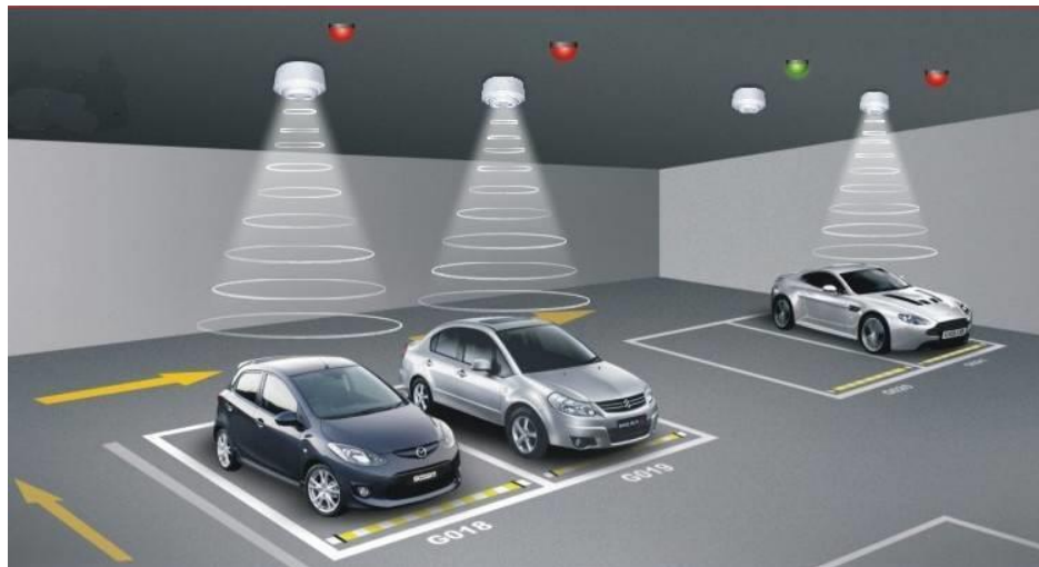
Figure 27: PGI system that implements LEDs with ultrasonic sensors to determine vacancy (Hiphen, .n.d)
