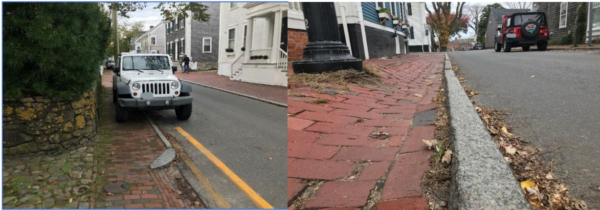
Figure 17: Sidewalk Parked Vehicle Obstructing Pedestrian Access & Damaged Sidewalk
