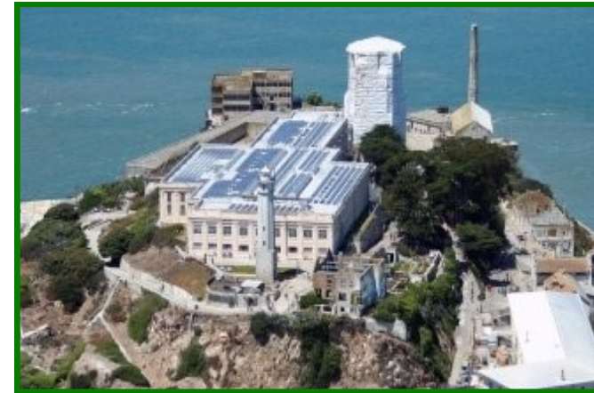
Figure 5. Alcatraz solar array (Office of Renewable Energy and Efficiency, 2017)
