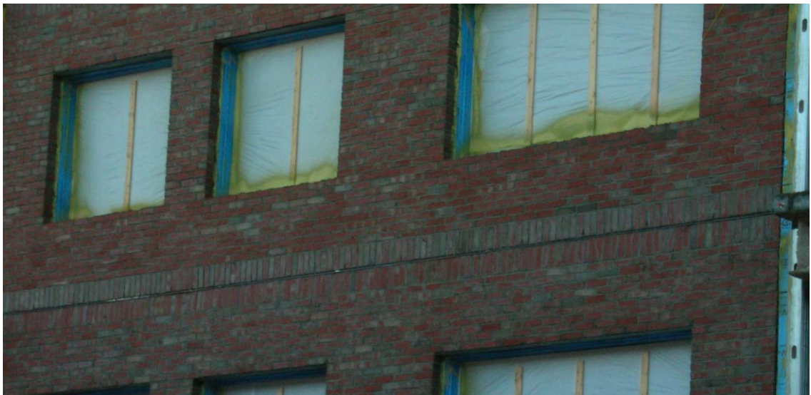
Figure 4: Running Bond and Solider Course
