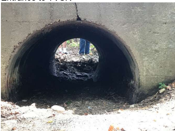
Existing Culvert under Snake River Road
