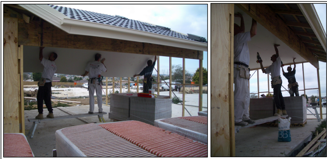
Figure 25 Fixing 6m plasterboard sheet to a ceiling
