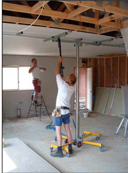
Figure 36 Fail-safe panel lifter in use with screw gun extension
