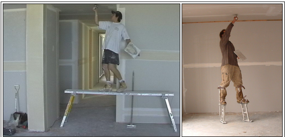
Figure 22 Hand trowelling of plasterboard joint
