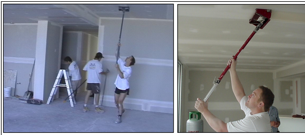
Figure 24 Trowel box in use
