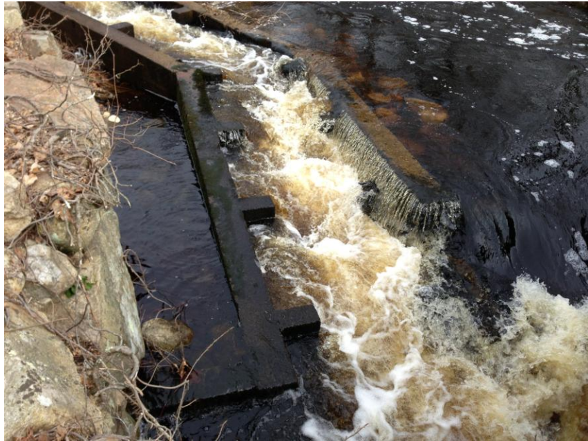
Figure 22: Weir-Pool Passage Under High Flows
