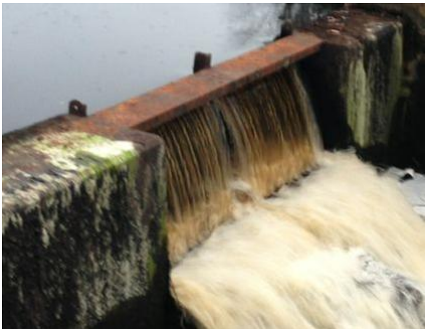
Figure 4: Russells Mills Dam
