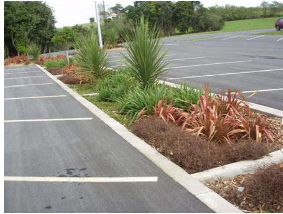
Figure 21: Bioretention Example 1 (Landcare Research, 2010)
