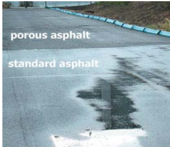
Figure 13: Permeable vs. Impervious Asphalt (Adams, 2003)
