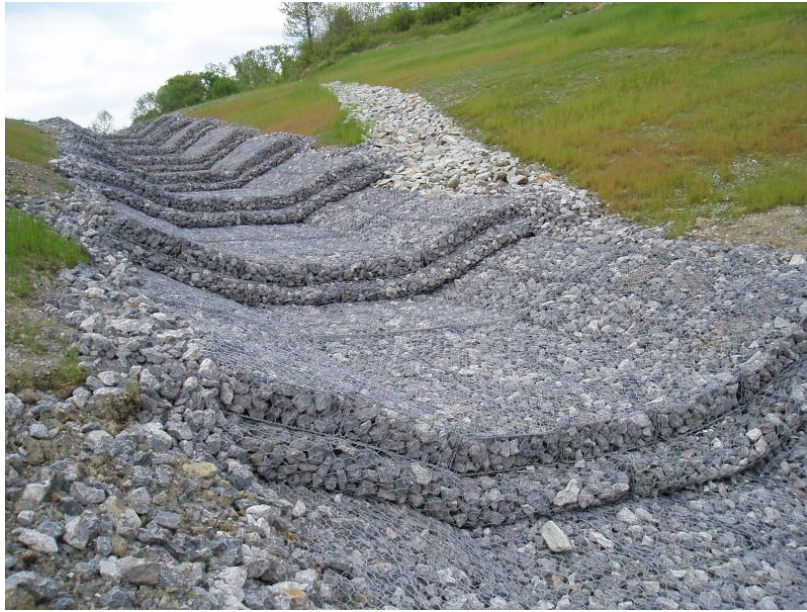
Figure 9 - Stabilization of slope area using gabions (South Fayette Conservation Group, 2008)
