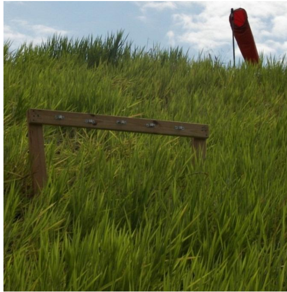
Figure 20 - Location of soil erosion bridge at site 5 showing hydroseeding (Photo Credit: Bryan Lee, 2011)
