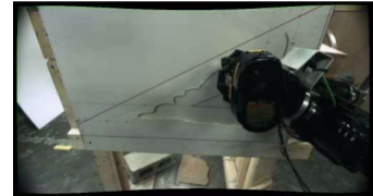
Figure 2.8: The front camera vision of drilling the wall
